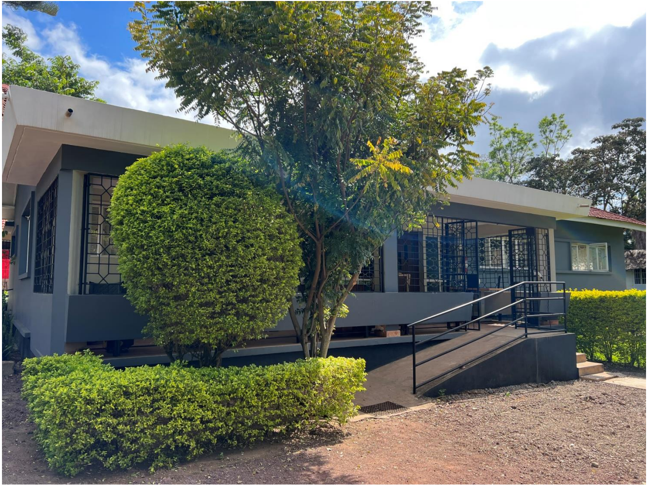
Front View of Miracle Experience Tanzania Limited's Office Building located on Plot No. 45 Block LDA located at Engira Road in Arusha City
