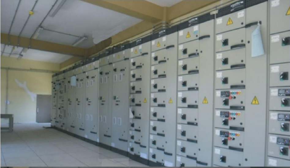
GREATER POLONNARUWA WATER SUPPLY PROJECT
