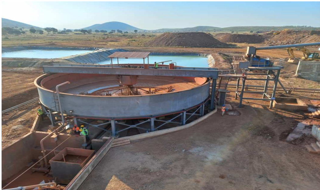
Fig. 1.3 - 2: Busolwa Gold Processing Plant at Ishokela - ML 555/2015
