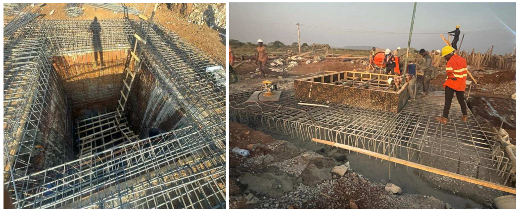
Fig. 2.1 - 1: Underground Shaft under Construction at the site
