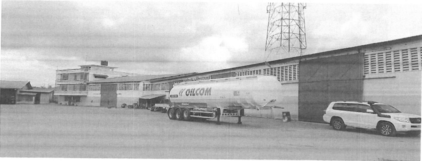
Warehouse for Trucks Spare parts
