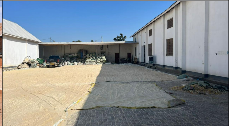
Existing milling plant and building
