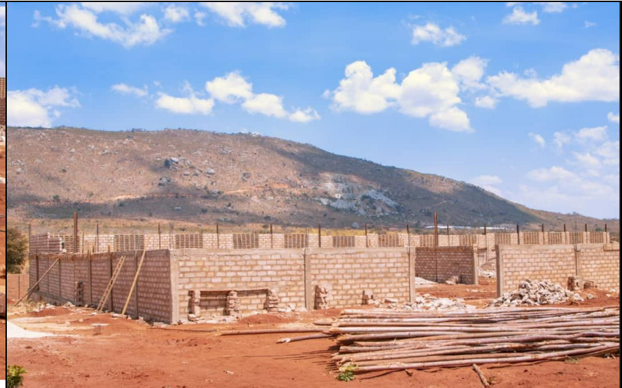
View of the ware under construction (Storage capacity 20,000MT)
