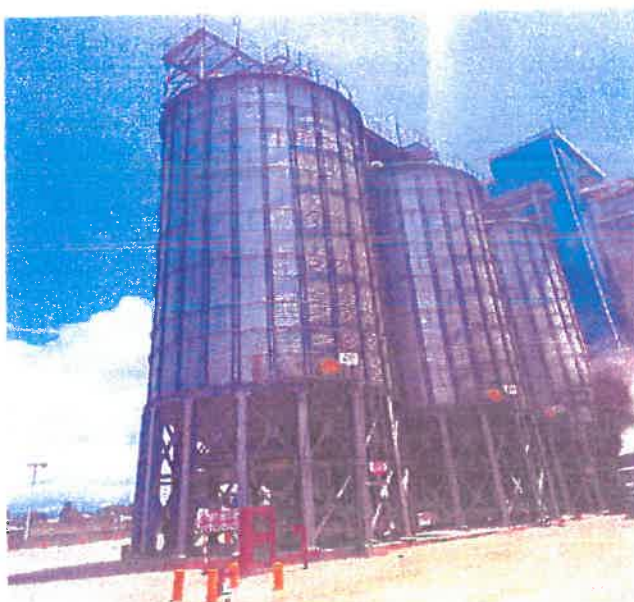
Expected look of the rice husk silos once construction is complete
