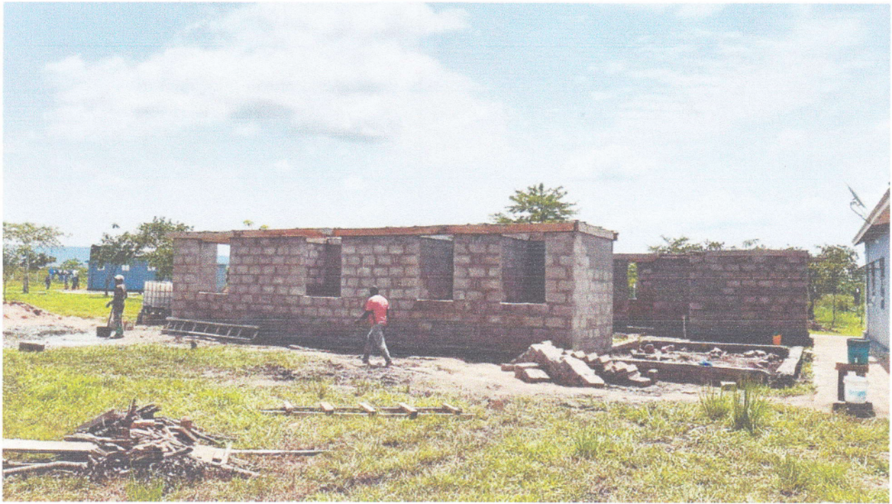
HOUSING ACCOMMODATION AND WORKSHOP IN CONSTRUCTIO
