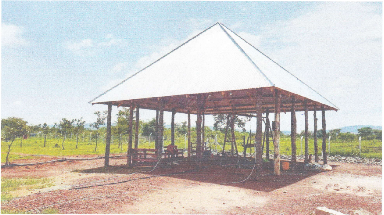
DEEP WATER WELL
