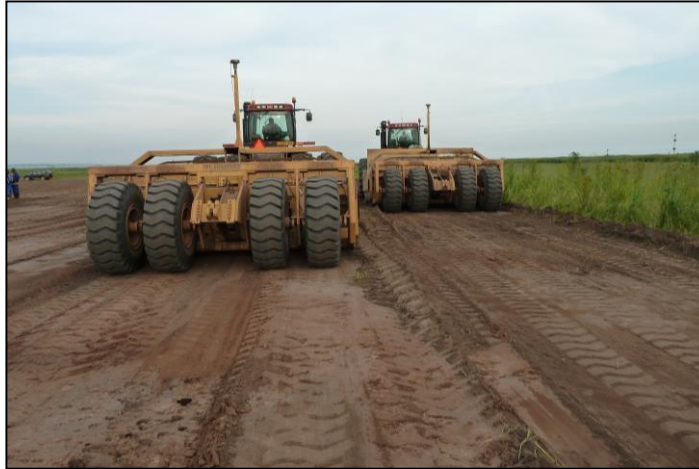
GPS controlled machine tractors and scrapers levelling the land
