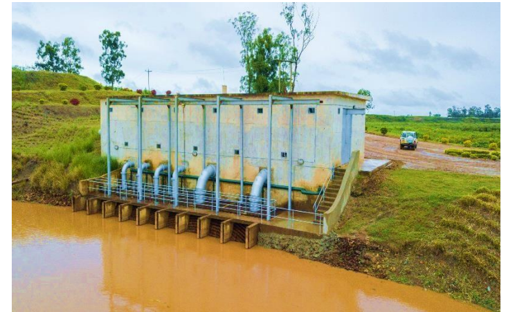
One of KSL's pump stations positioned at the Kagera river
