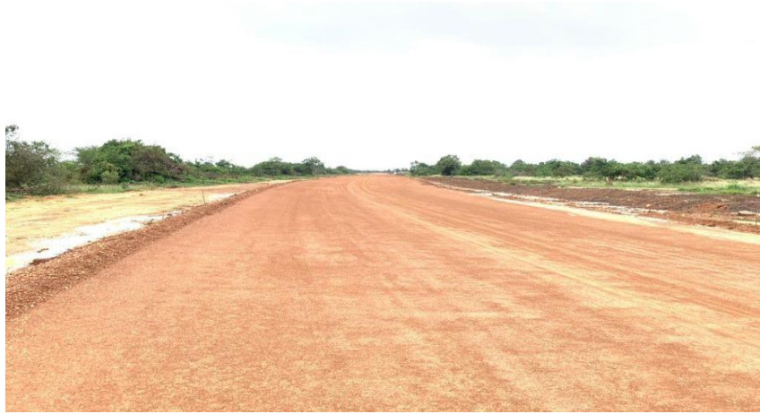
Ongoing construction of road infrastructure that connects to the bridge.
