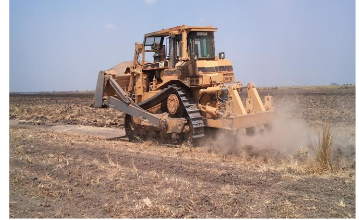
Step 2/3: A second clearing process to knock down the anthills, Ripping and initial levelling of the land
