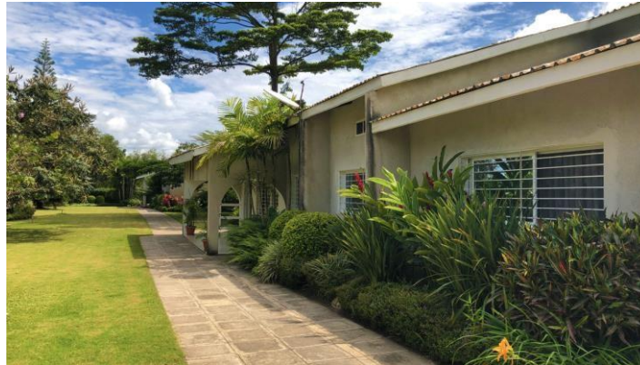
One of the types of staff houses built on KSL's estate.
