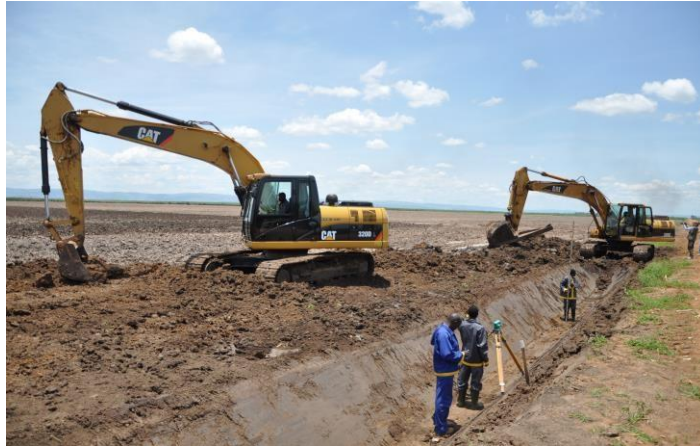
Step 7: Installation of drainage system to irrigate the cane effectively.
