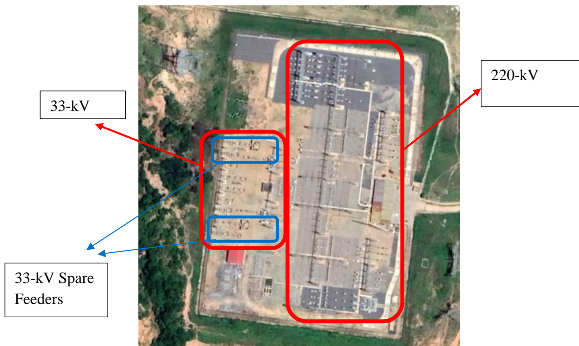
Figure 15: Status of the TANESCO Substation for the locations identified from the general layout (Source: AFA and Google Earth)
