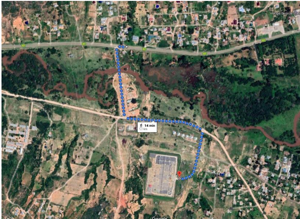
Figure 14: TANESCO Substation Access Road (Source: AFA and Google Earth)
