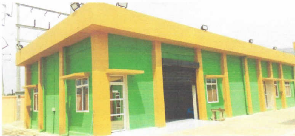
Front view of the switch yard building
