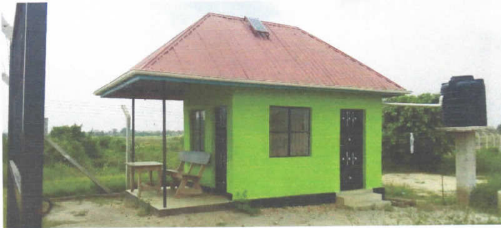
Front view of the outbuilding II
