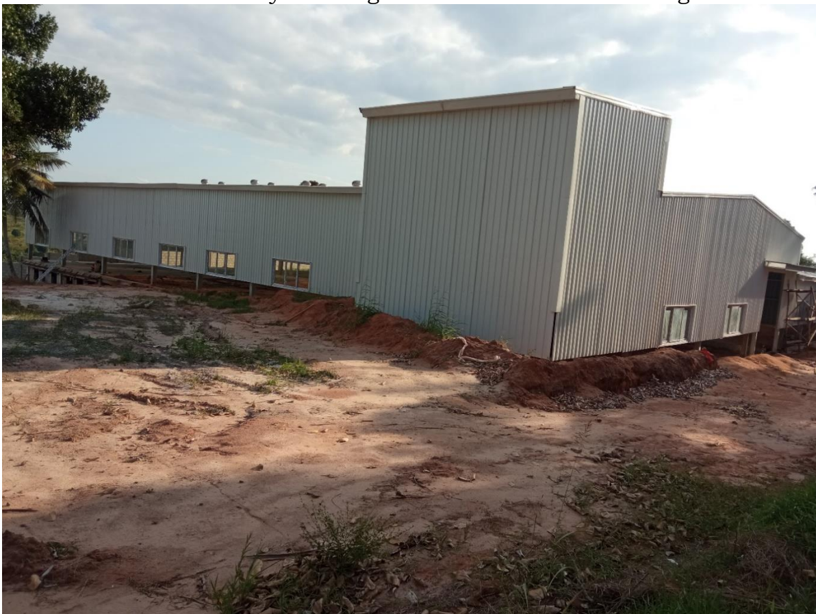
Factory Building Painting wings
