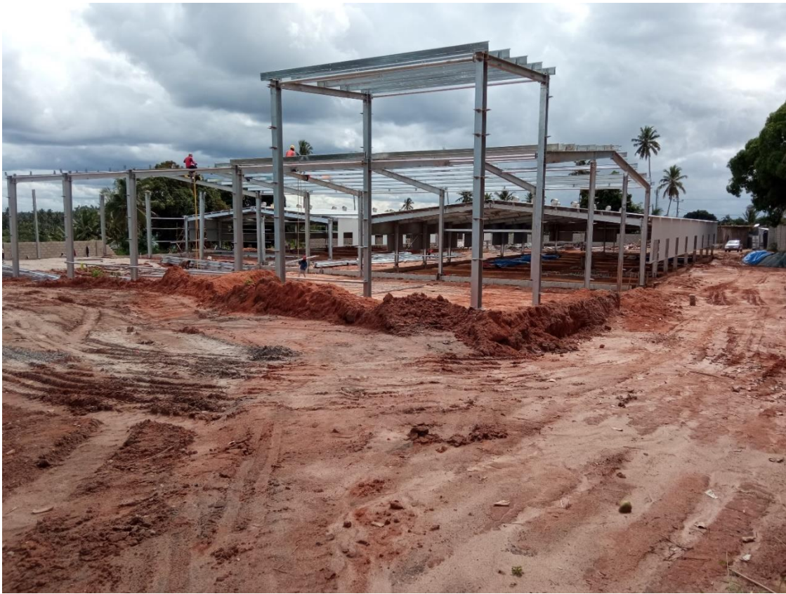
Factory Building on different contraction stages
