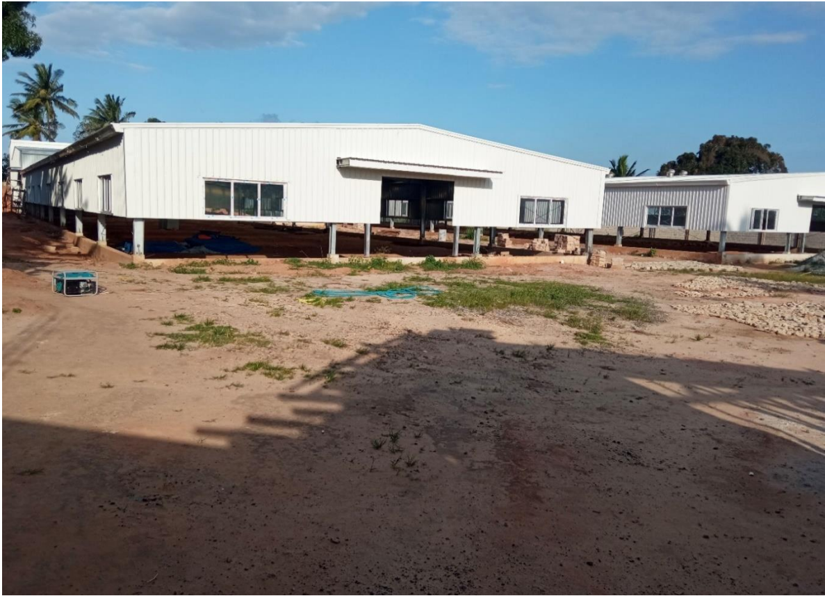
Factory Building; Wings A & B For Machinery & Storages Respectively
