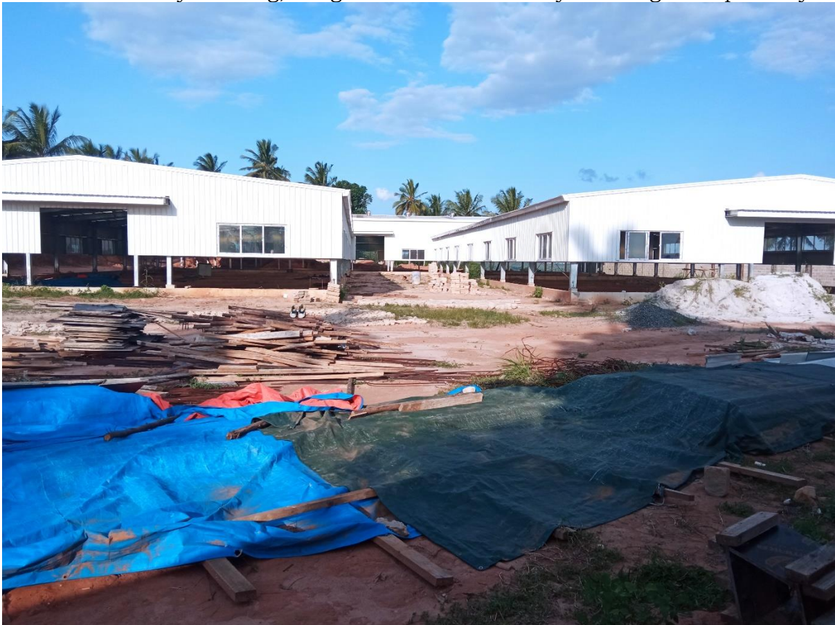
A Complete Factory Structure on finishing stage
