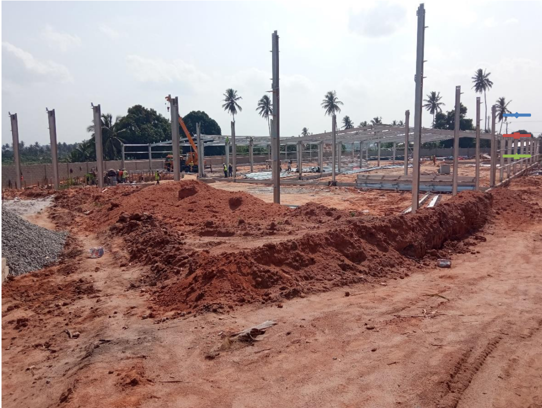
Factory Buildings at early stage of constructions
