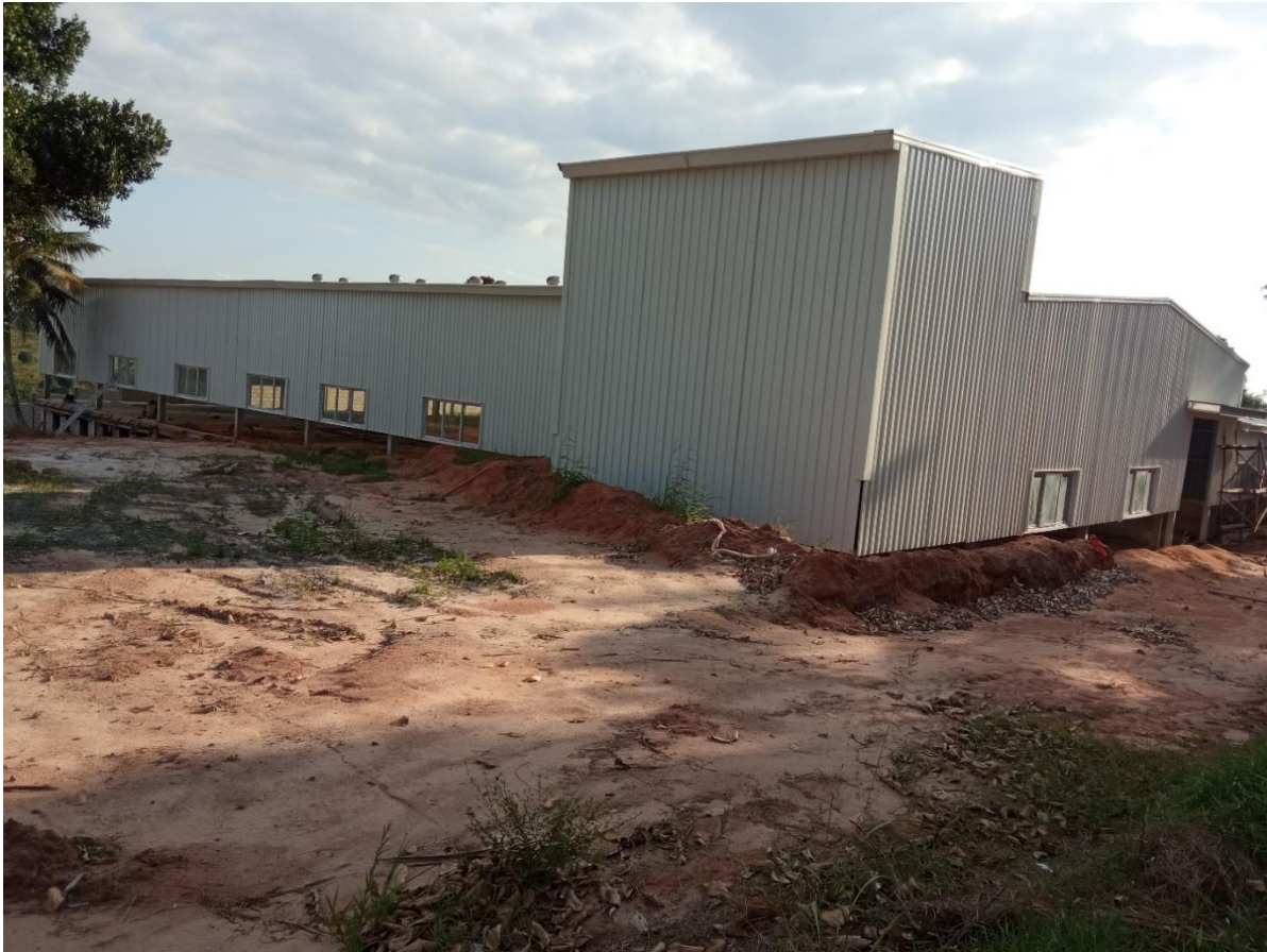
Factory Building Painting wings
