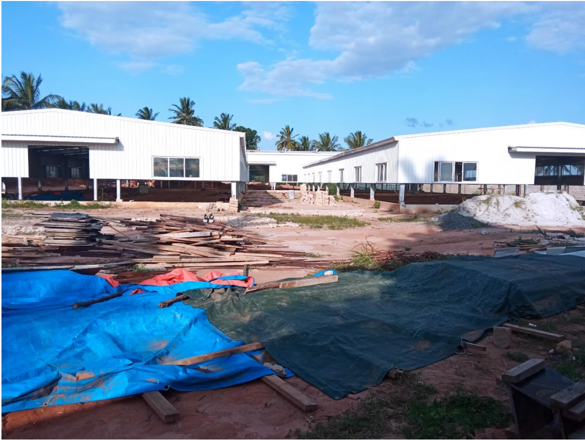
A Complete Factory Structure on finishing stage
