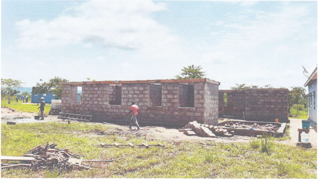
HOUSING ACCOMMODATION AND WORKSHOP IN CONSTRUCTIO
