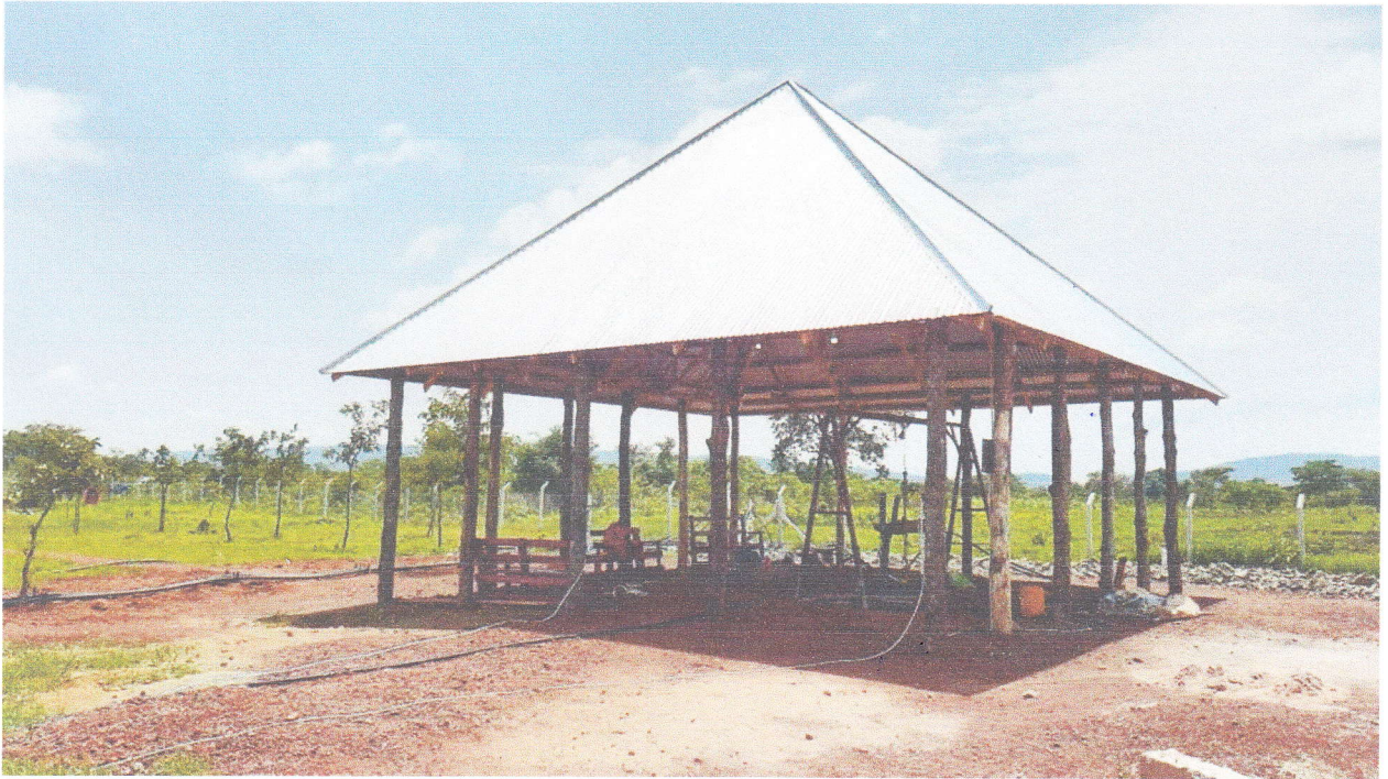
DEEP WATER WELL
