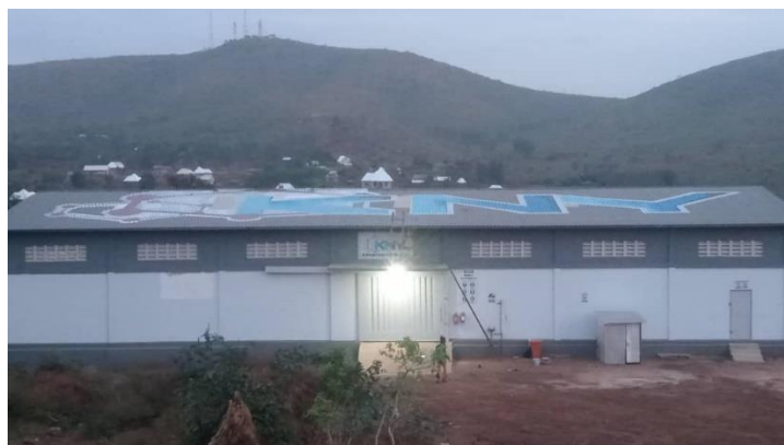
Warehouse in Geita (550 Square Metres)
