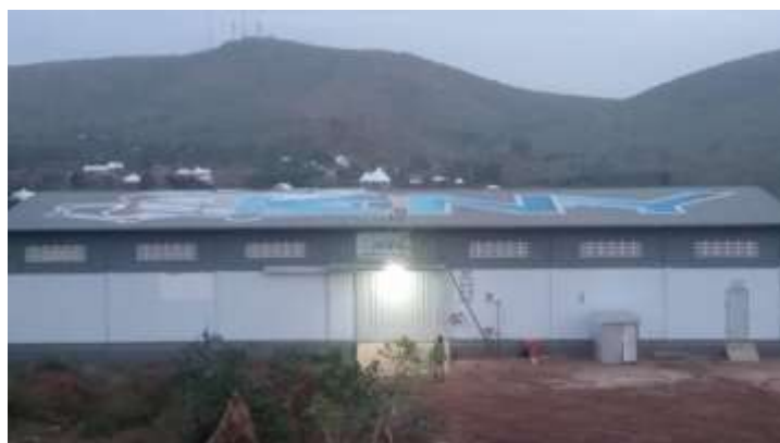
Warehouse in Geita (550 Square Metres)
