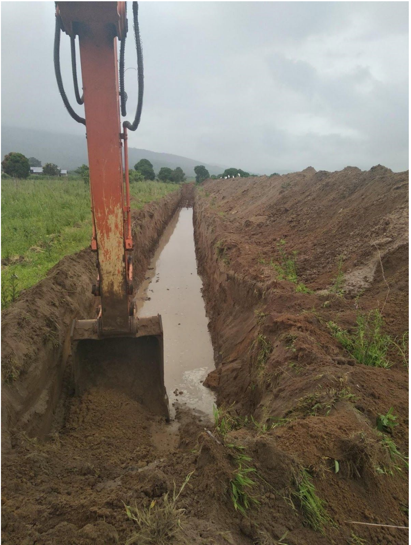
Boundary Trenching Around the Farm
