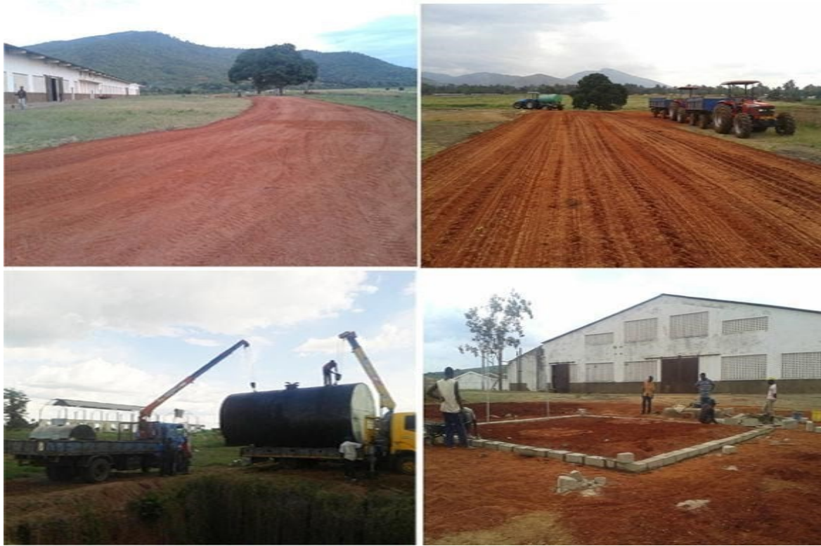
Erection of Fuel Station and Roads Formation
