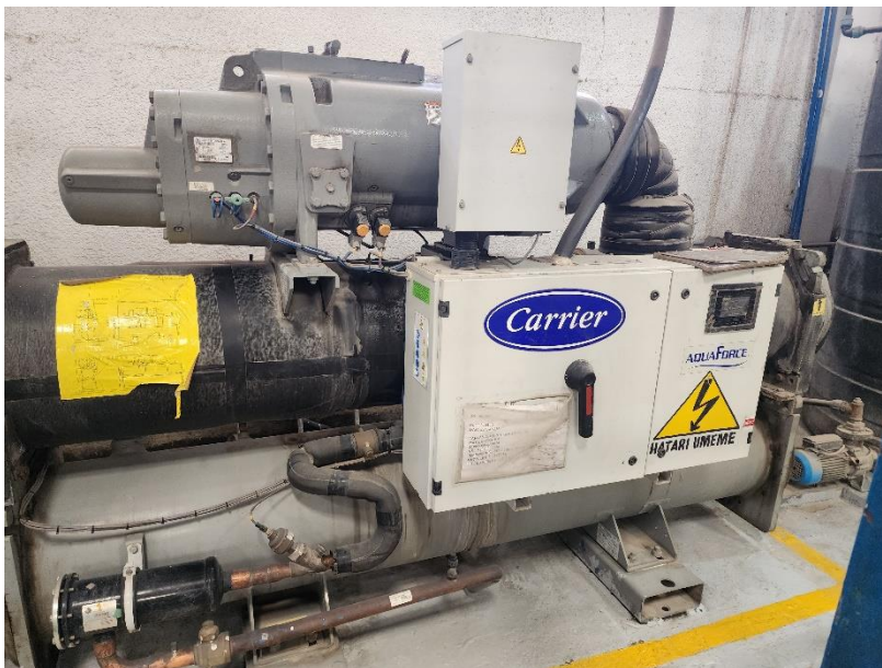
7) INDUSTRIAL SCREW WATER CHILLER (499 kw)
