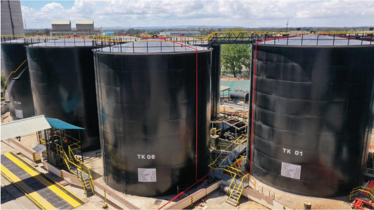
PICTURE 2: FULE BULK STORAGE UNDER CONSTRUCTION
