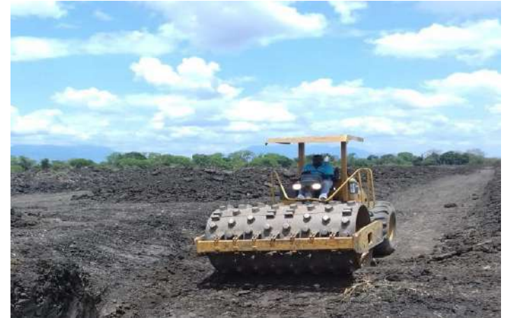
Ongoing work at the dam
