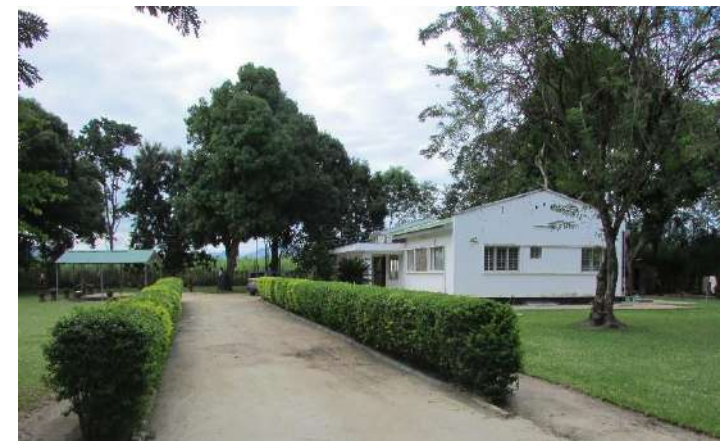
Photo: Renovated house at MSE's estate
