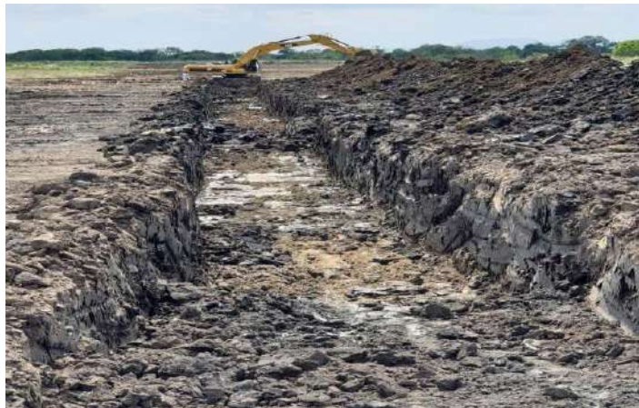
Construction of Dakawa dam 2
