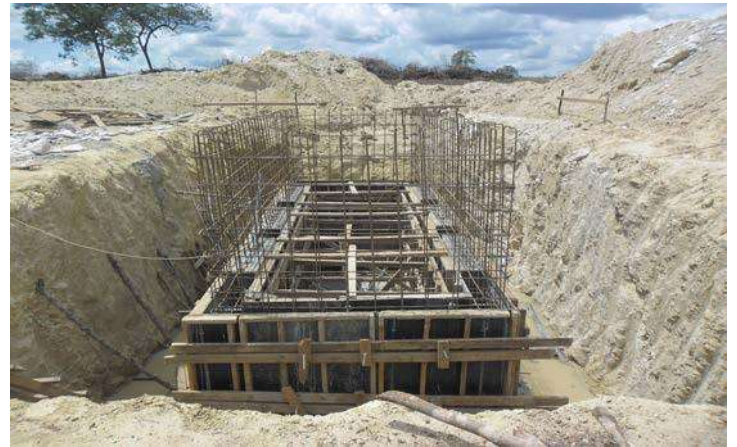
Building of a pump station at Dakawa
