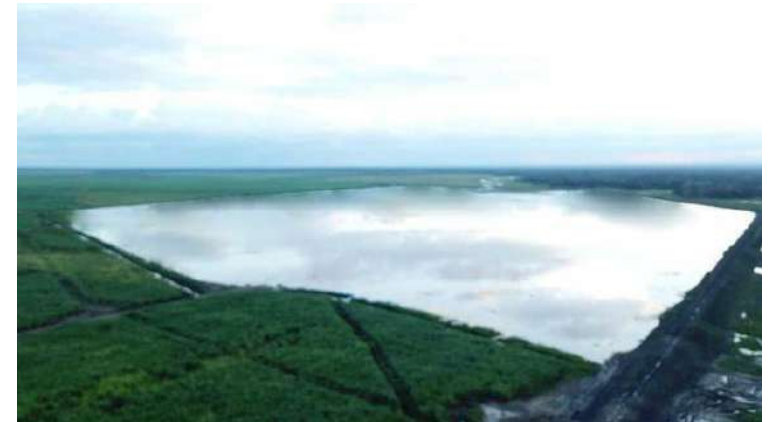
The B4 dam on Dakawa 1 farm at MSE.
