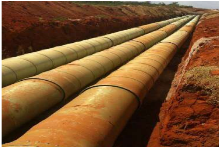
Installation of water pipes as part of the irrigation infrastructure.
