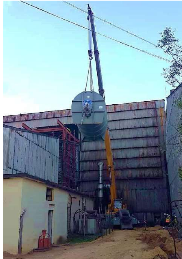
Ongoing factory expansion
