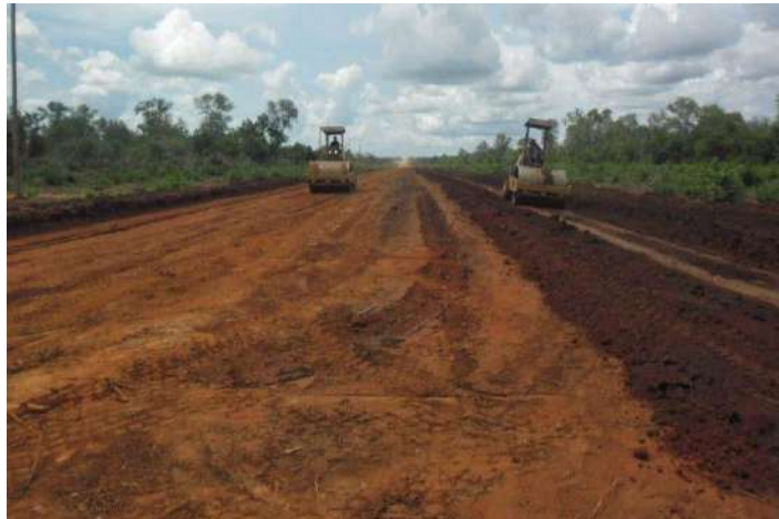
One of the roads constructed by MSE.
