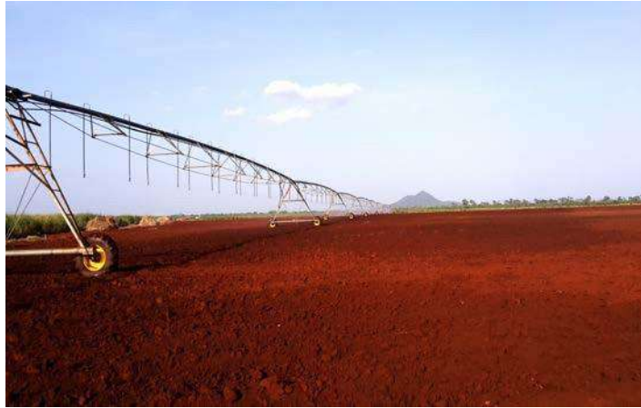
Installation of centre pivot irrigation structure.
