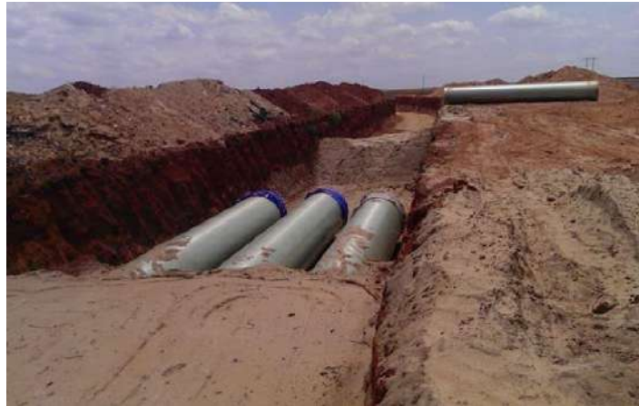
Step 7: Installation of main water pipelines.
