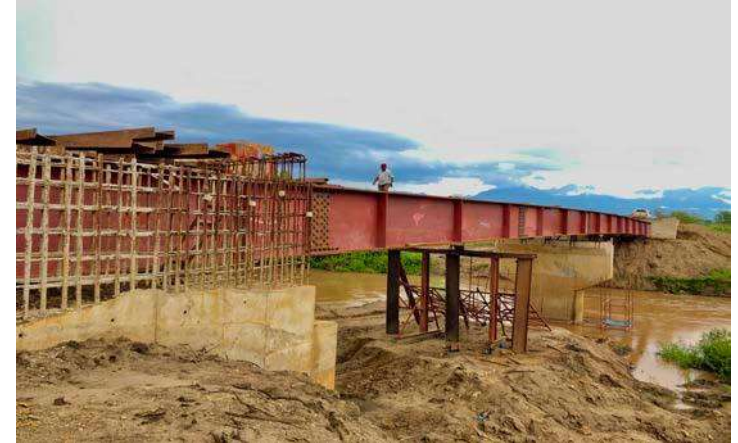
New bridge under construction.
