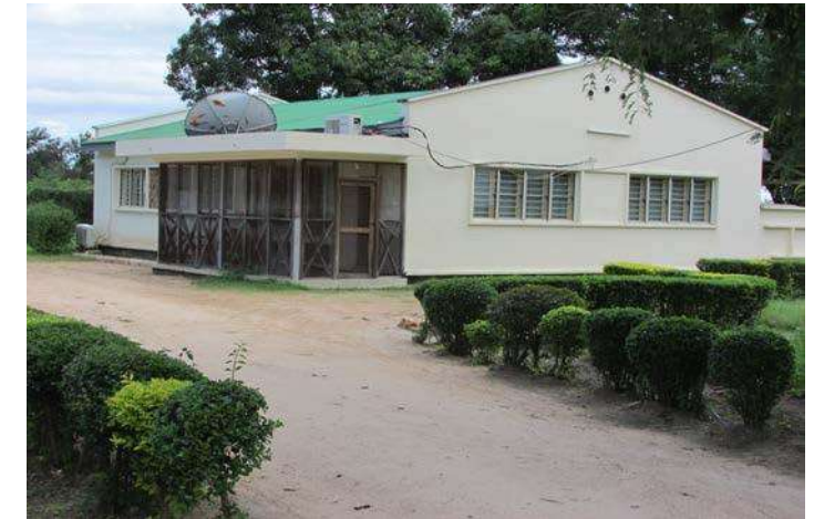
One of the refurbished houses at the MSE estate.
