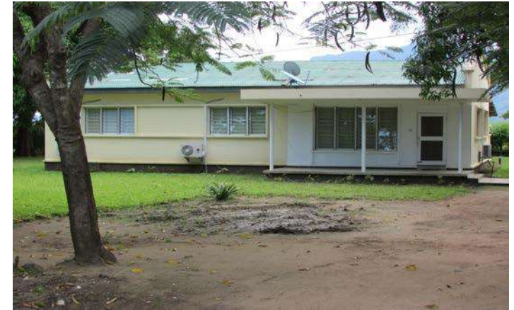
Photo: Renovated house at MSE's estate
