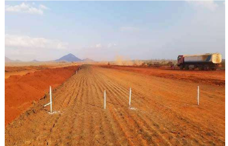
One of the roads constructed by MSE.
