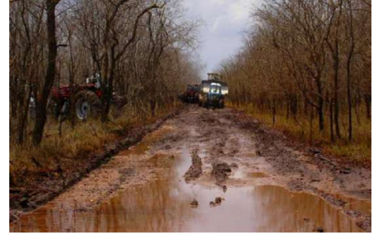
MSE faced challenges using the existing road network especially during rainy seasons.
