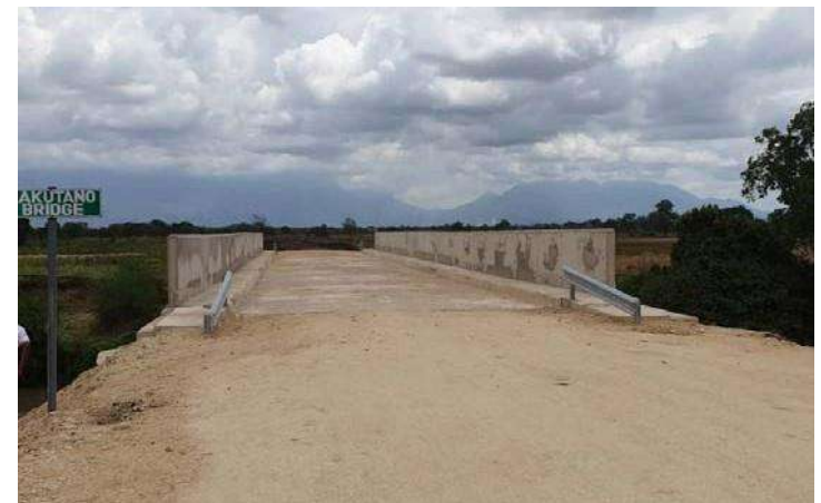
New bridge over the River Wami
