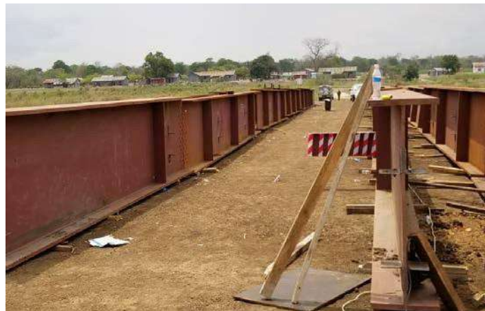
New bridge under construction.
