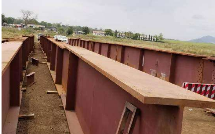
New bridge under construction.
