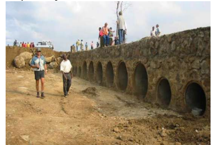
Temporary bridge installed over the River Wami
