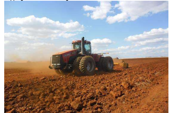
Step 5/6: GPS controlled machine tractors and scrapers levelling the land, followed by ripping operation
