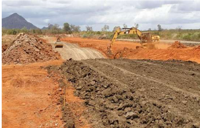
Construction of a dam wall
