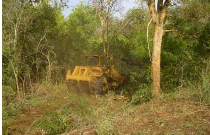
Step 1: Initial clearing of shrubs and trees on an undeveloped land
