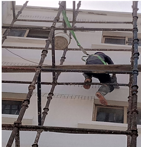
B05, Cutting cracks between wall and beam
