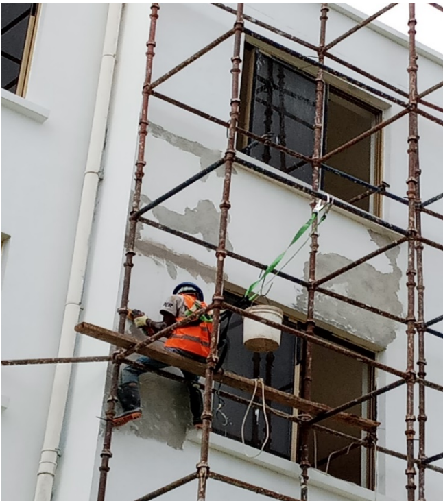
B09, Fixing plumbing appliances
