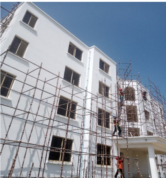
B06 , Removing external scaffolding work
