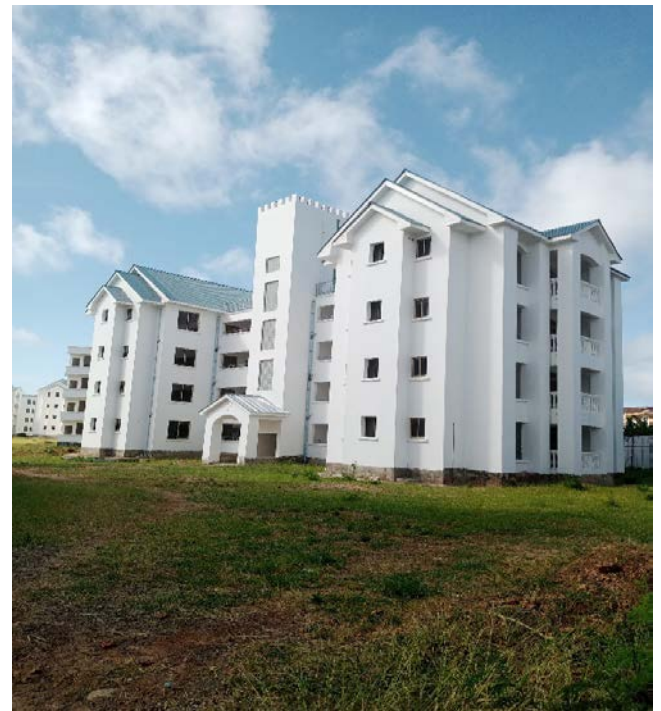
B01, Cracks plaster repair work
