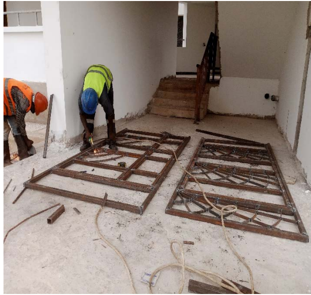
B11, MS entrance double and single door making
