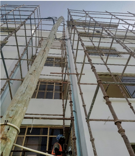
B06, external skimming work
