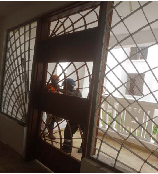
B11 , Fixing MS entrance single door work
