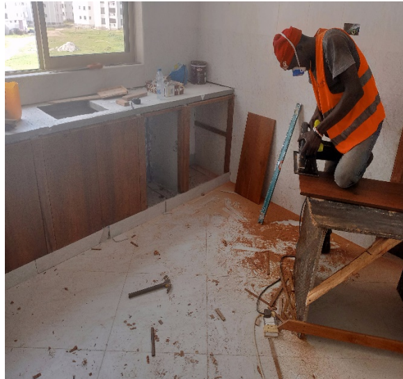
B02, SF kitchen cabinet fixing work
