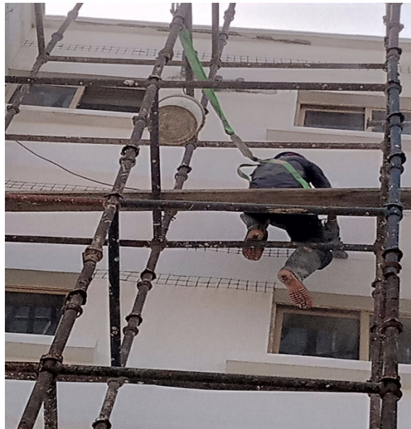
B05, Cutting cracks between wall and beam
