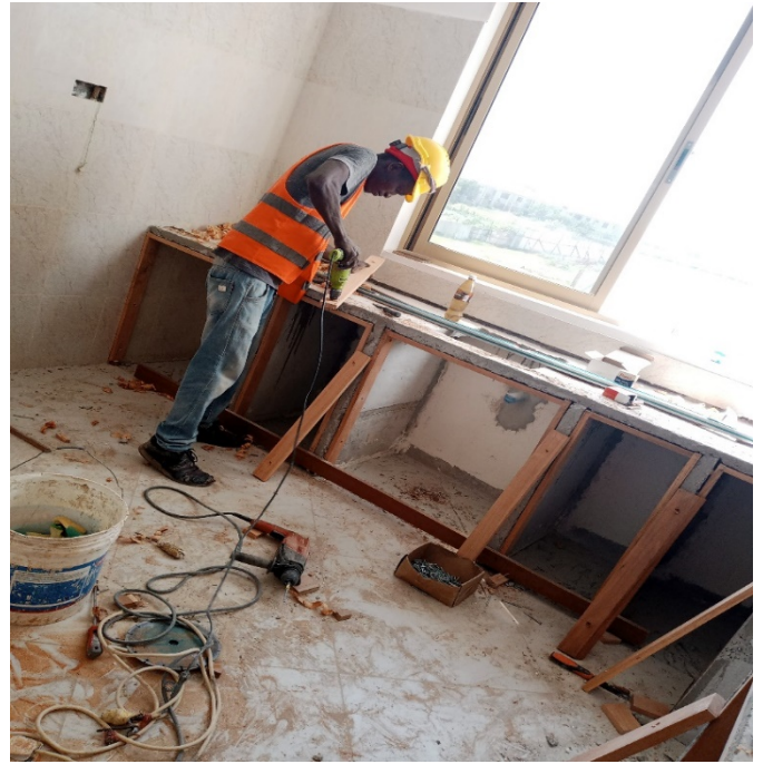
B03, Kitchen cabinet fixing work
