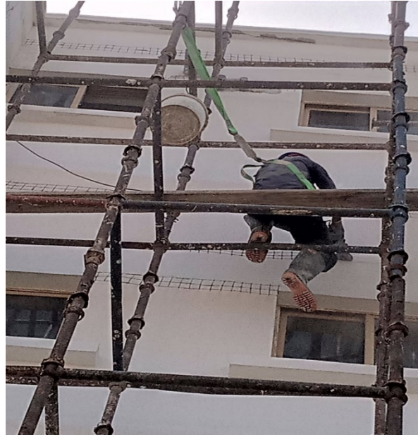
B05, Cutting cracks between wall and beam
