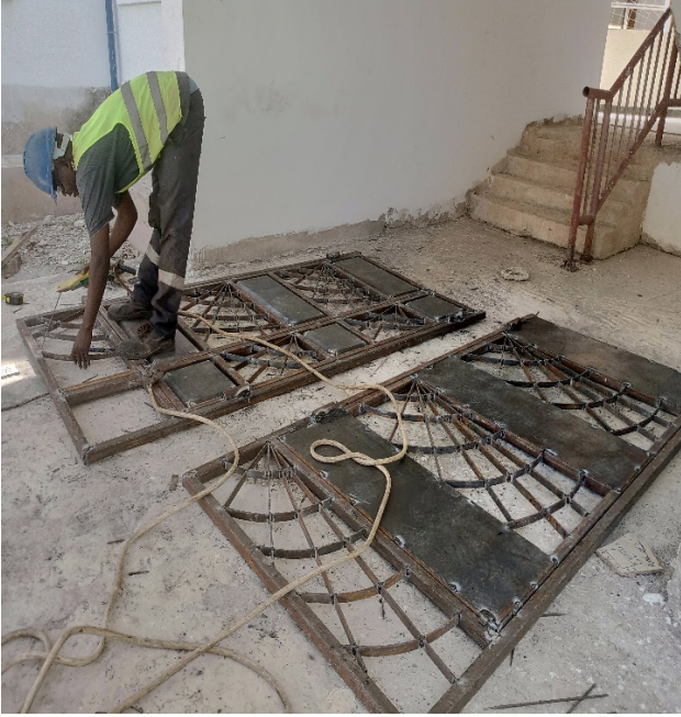
B11, MS entrance double & single door making work
