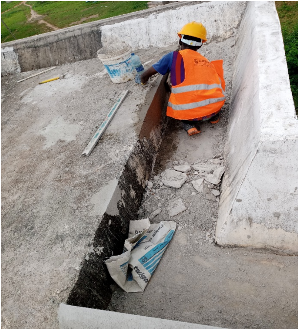
B01, Roof slab rain gutter cleaning work
