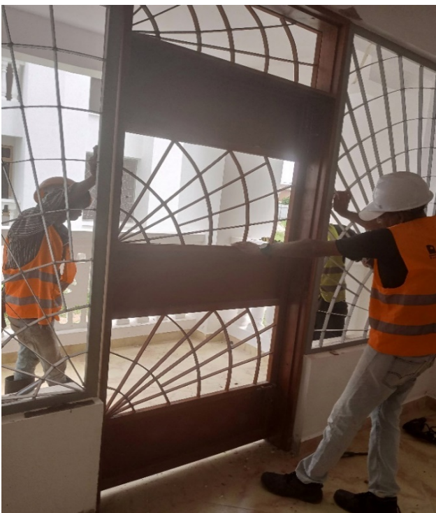
B10, Fixing MS entrance door
