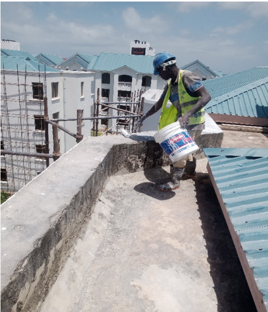
B05, Parapet wall primer painting work
