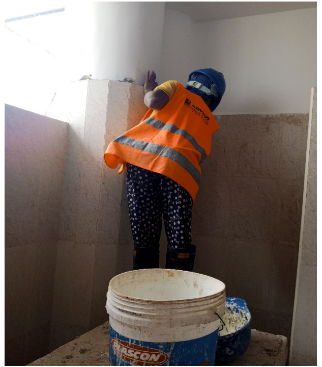
B01, Toilet Wall grouting work
