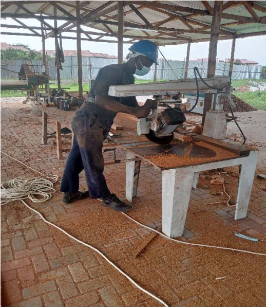
W/shop, B09 & 10 Ducts door flames making
