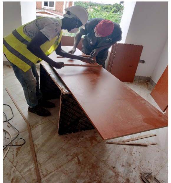
W/shop, kitchen cupboard making work
