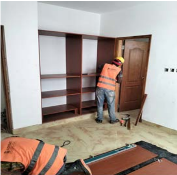
Building No. 03, wardrobe fixing work is under progress
