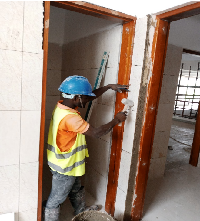
B01, Toilet wall tilling work
