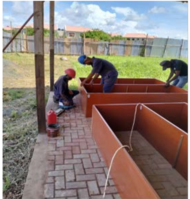
B03, wardrobe making work is under progress
