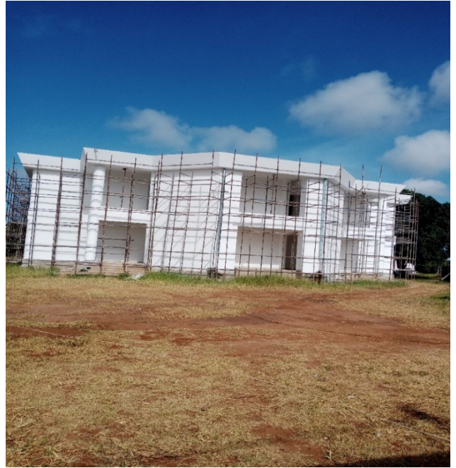
B01, Left side scaffolding
