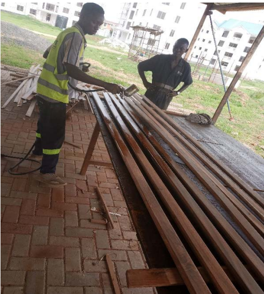
W/shop B08, Archtraves painting work work
