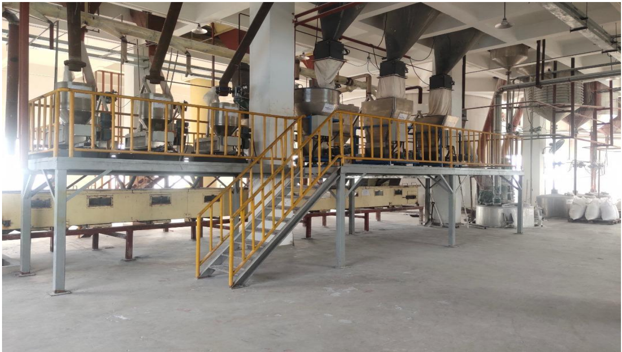
Picture No.8 Washing powder manufacturing machines workshop
