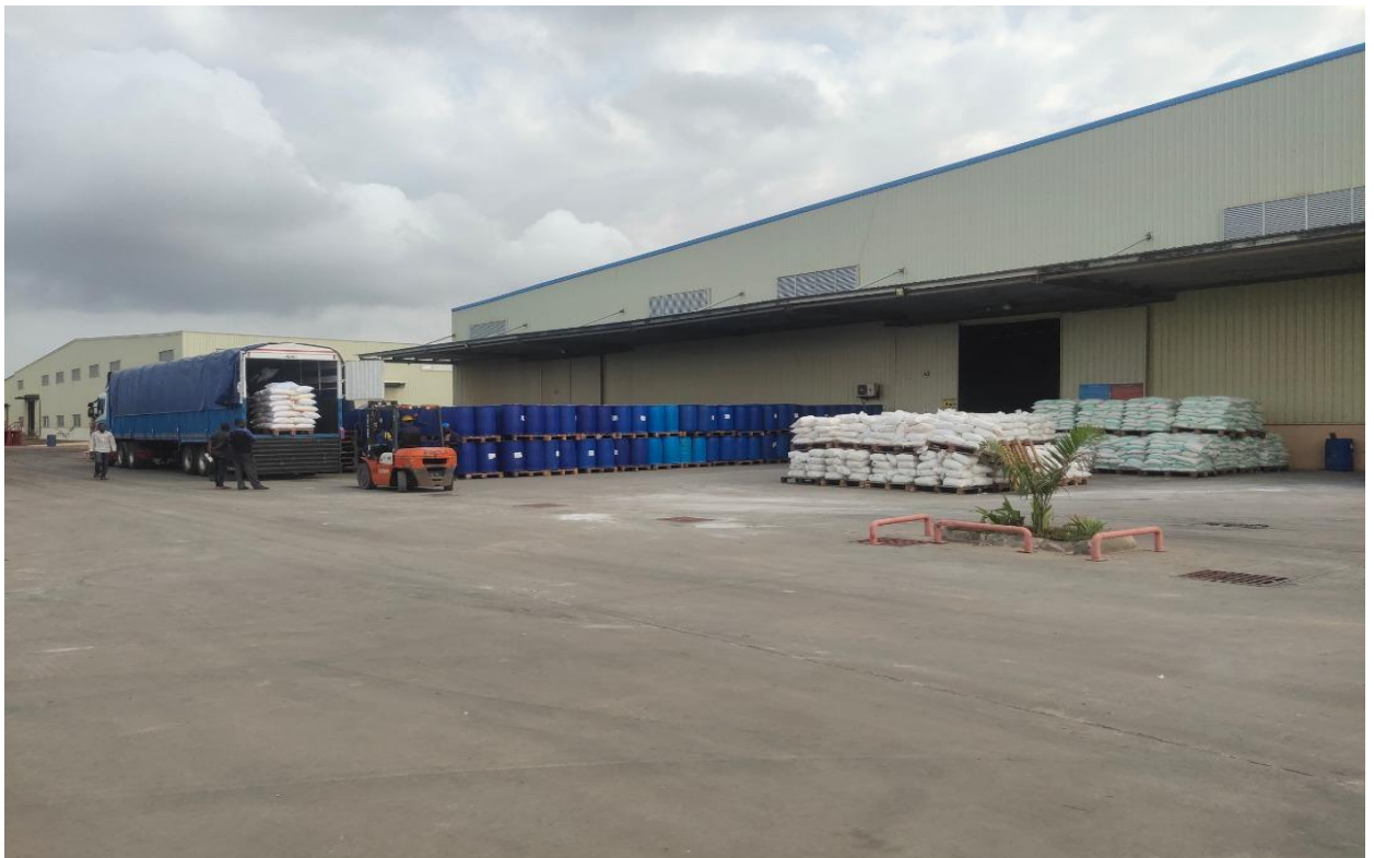
Picture No. 11 Outside Washing powder warehouse
