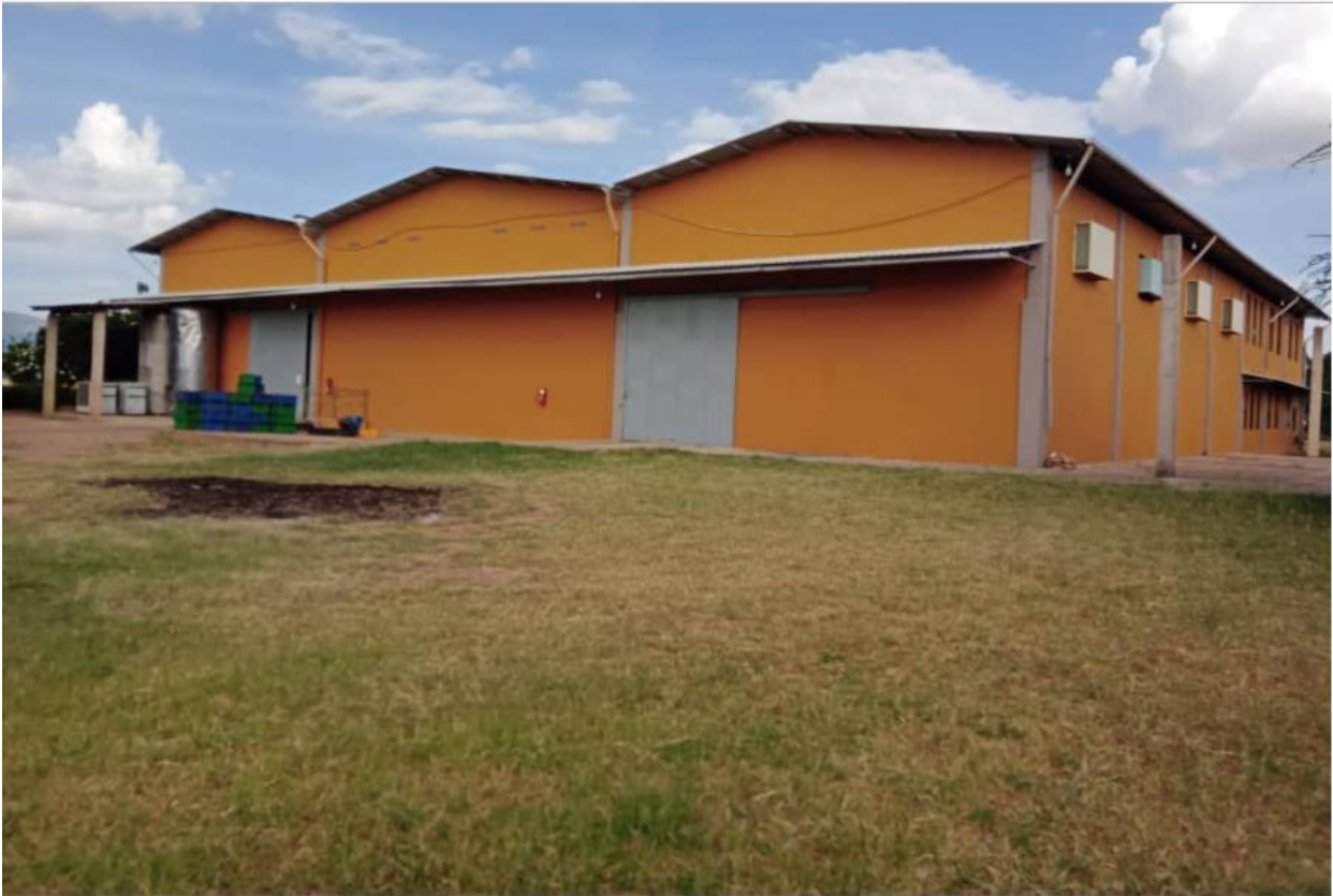
After renovating back side view
