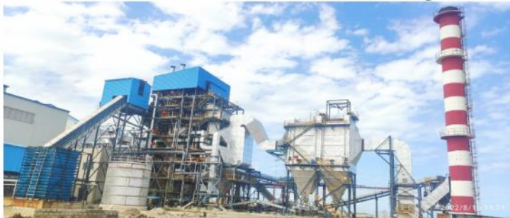
Present Status – After completion
