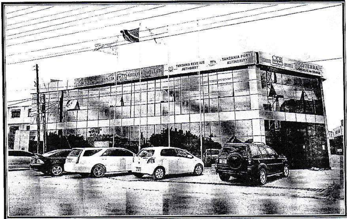
PMM'S HEAD OFFICE AND ICD YARD
