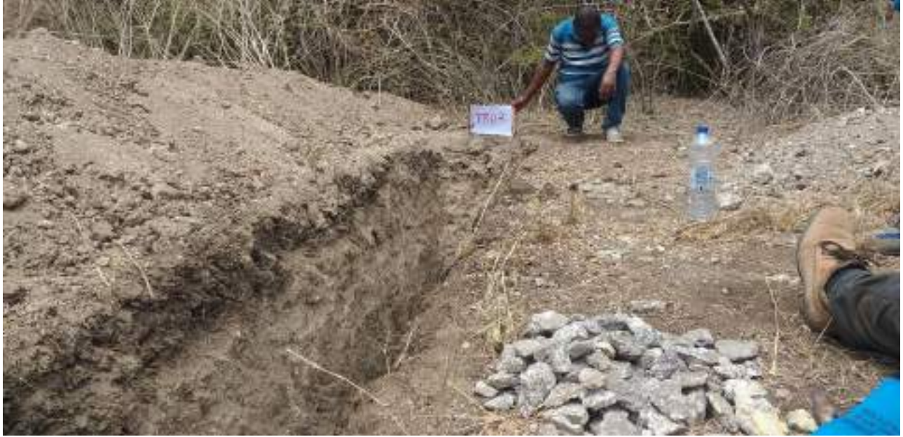
Plate 2.8 Weathered graphitic gneiss exposed from trench number 09, Kwamsisi Graphite Project, Handeni 风化石墨片麻岩从 09 号沟中暴露出来 (Source: Azustone Resources (T) Ltd, field work, 2022)
