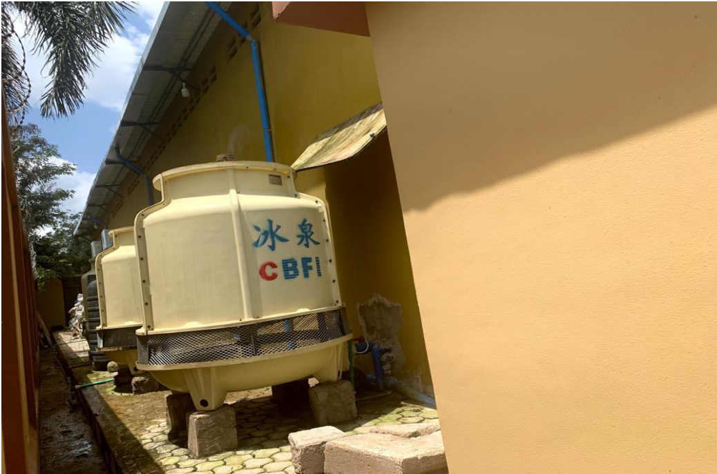
Water Reserve Tanks
