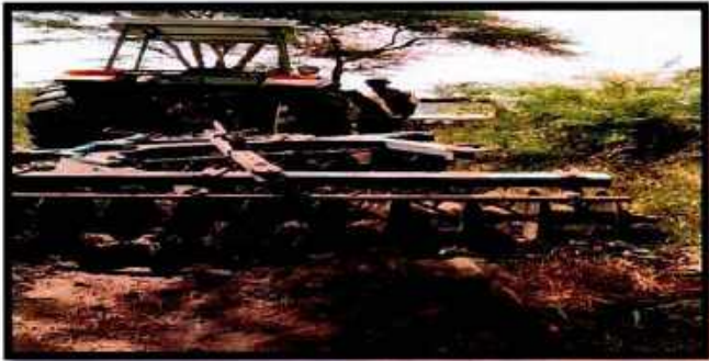
Picture 9: A company tractor undertaking road construction in Maswa GR.
