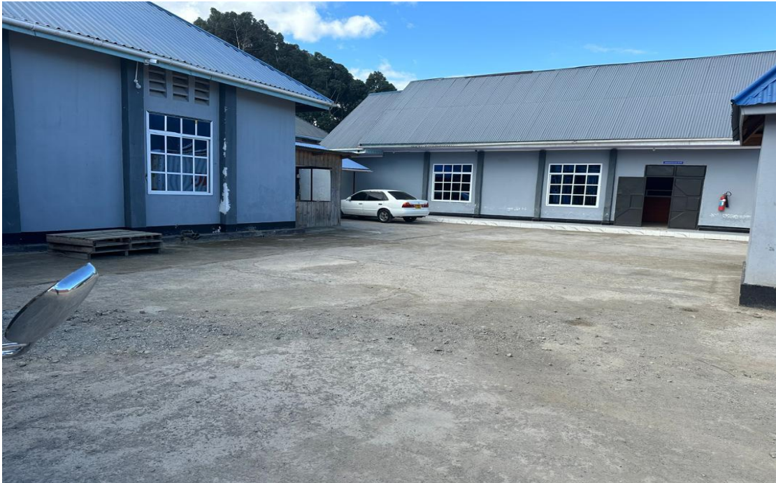
Warehouse where machinery is installed and production takes place
