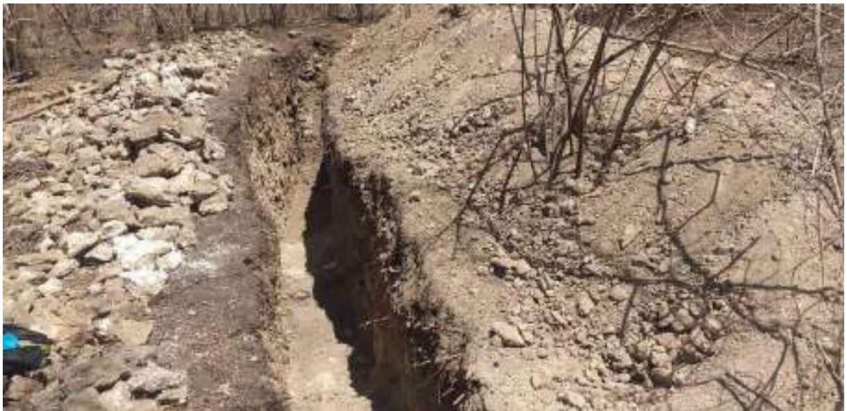
Plate 6.3: Trench Number 5 (TR05), crosscutting graphite mineralised weathered crystalline limestone, Kwamsisi Graphite Project, Handeni.
