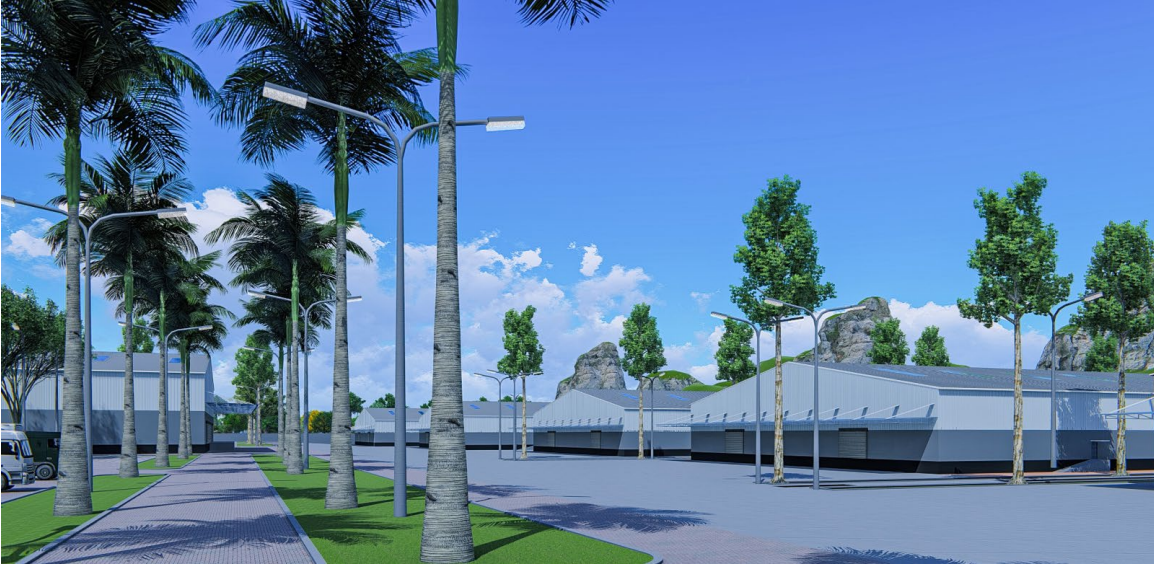
Mwenge Industrial Park
