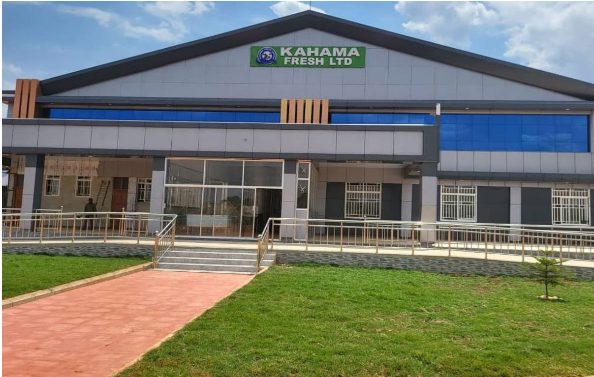
Figure 3: Kahama Fresh Ltd Constructed Building for the Milk Processing Plant- Front view
