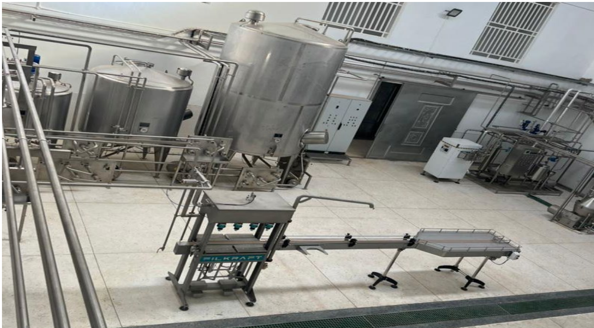
Figure 6: Installed Yoghurt Processing Unit
