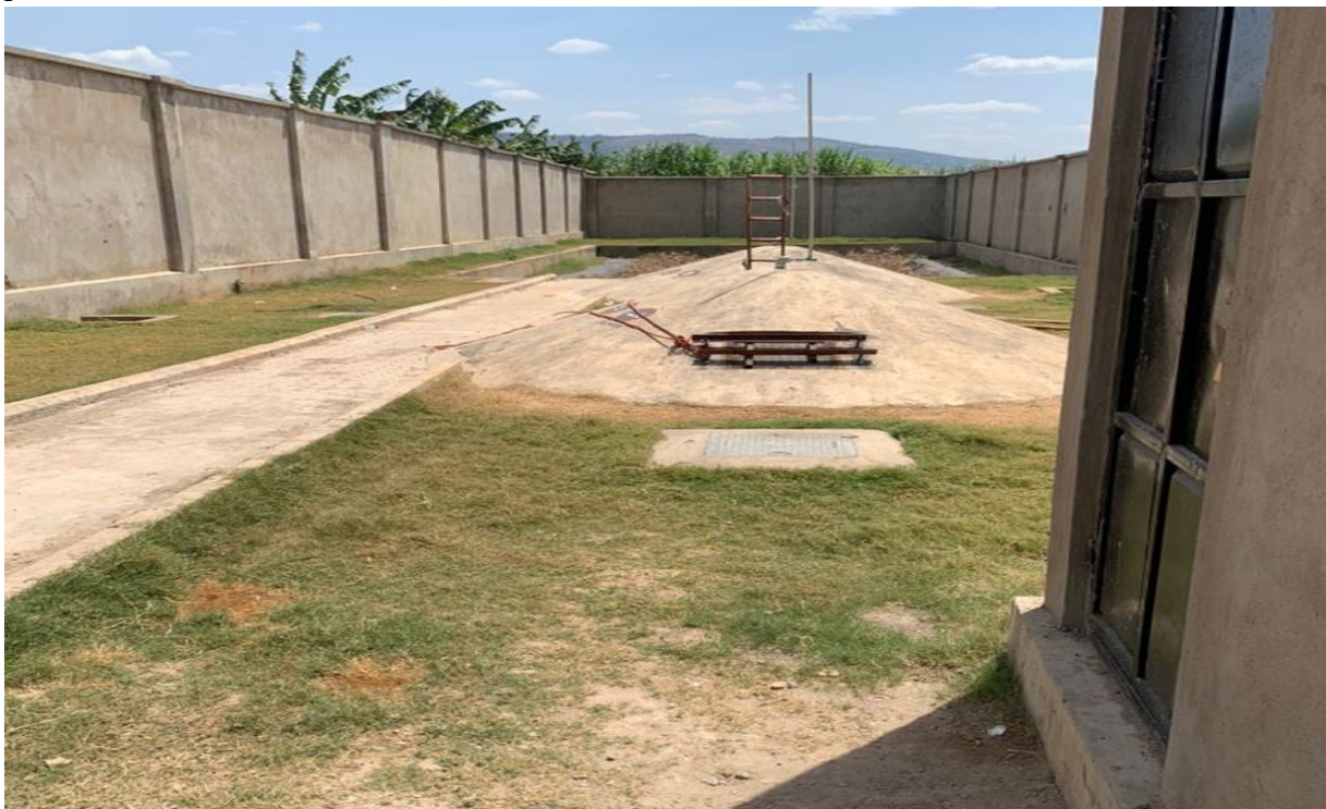
Figure 10: Constructed Water Well at Ranch
