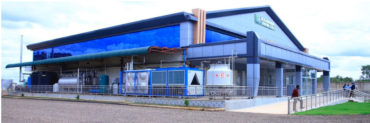
Figure 1: 20,000 LTRS Milk Processing Plant Installed at Karagwe, Kihanga Industrial (Side View- Utilities section)
