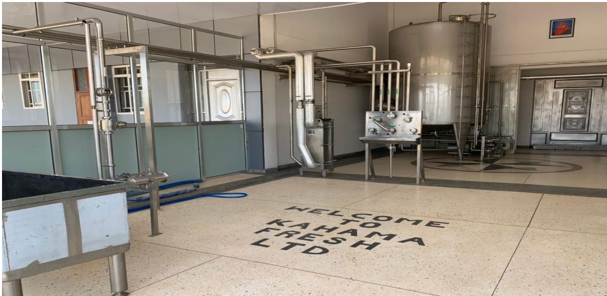
Figure 9: Raw Milk Receiving Point at the factory (Sideview section)
