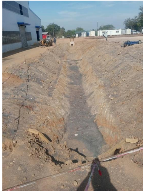
Photo 17. Storm water trenches around the plant area
