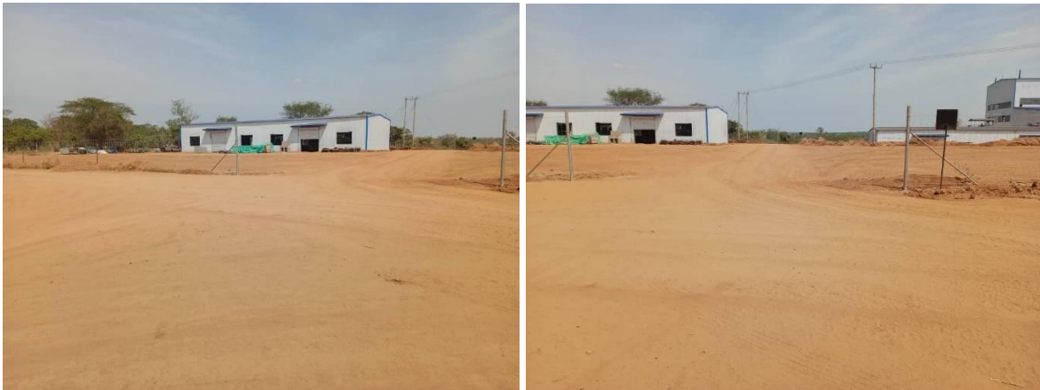
Photo 16: Plant access roads trimmed and compacted well around main entrance gate & warehouse
