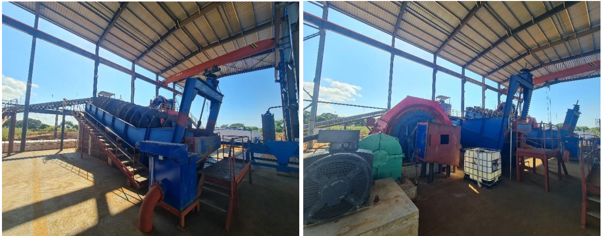
Photo 7: Scrubber, road and pebble mill at Lindi Jumbo Mine Site during commissioning
