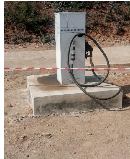
Photo 18. Fuel storage and dispensing facility at plant area
