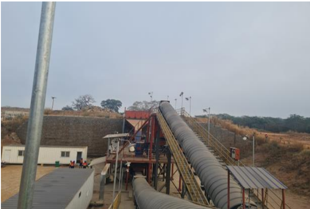
Photo 6: ROM bin, liners and feeders belts at Lindi Jumbo Mine Site
