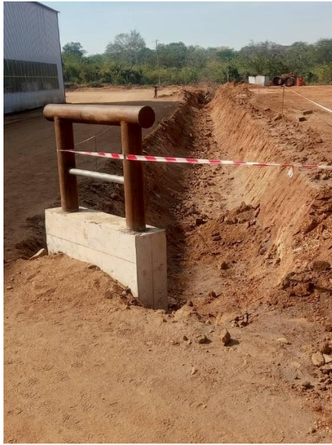
Photo 17. Storm water trenches around the plant area
