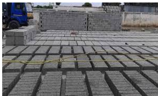
Curing step in Concrete block and paver manufacturing
