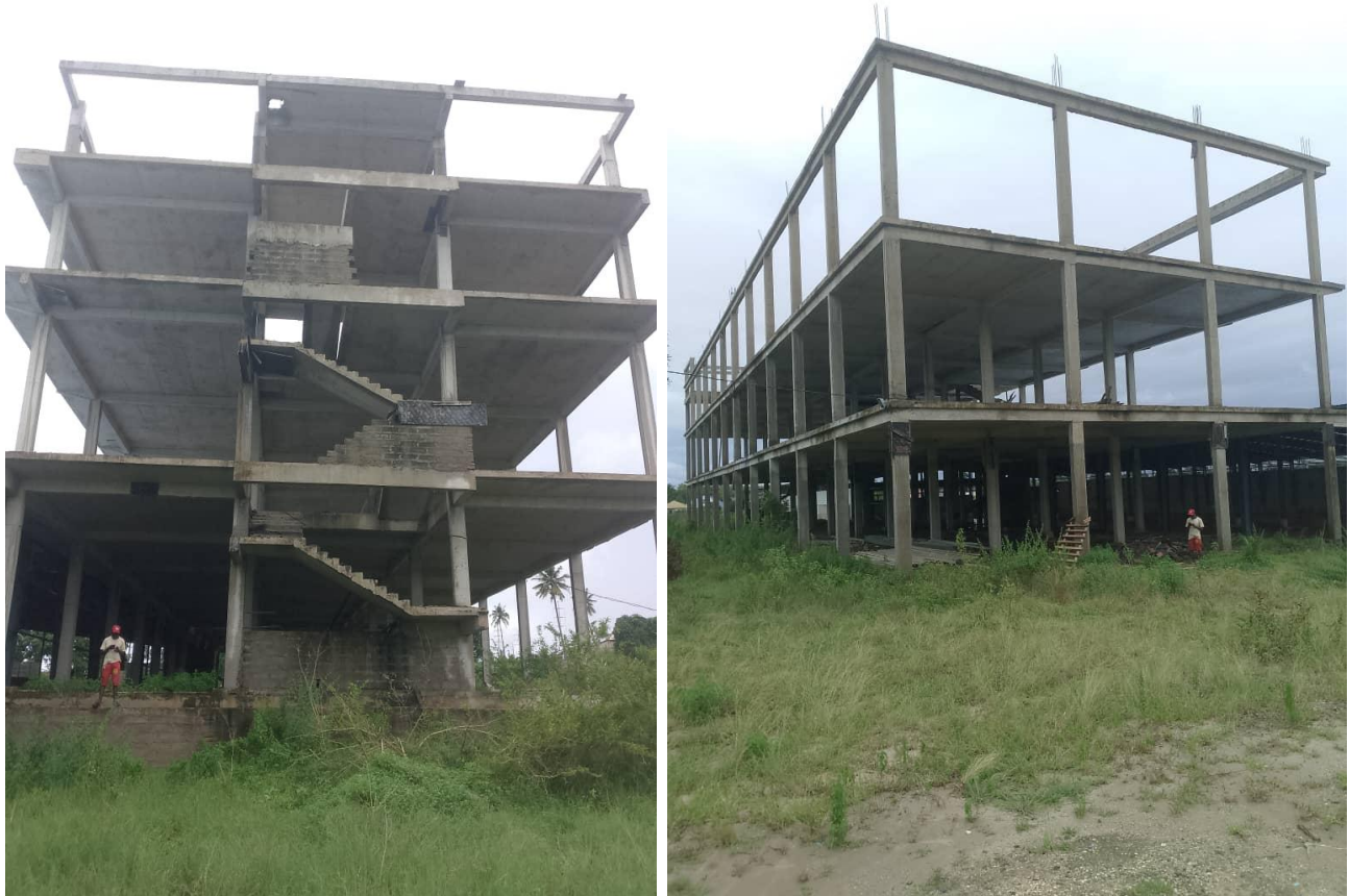
Photos showing the concrete framed structure of an office building.
