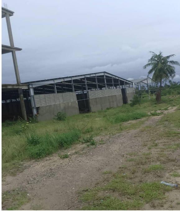
Photo showing the steel columns, beams, trusses and purlins erected at the warehouse buildings.
