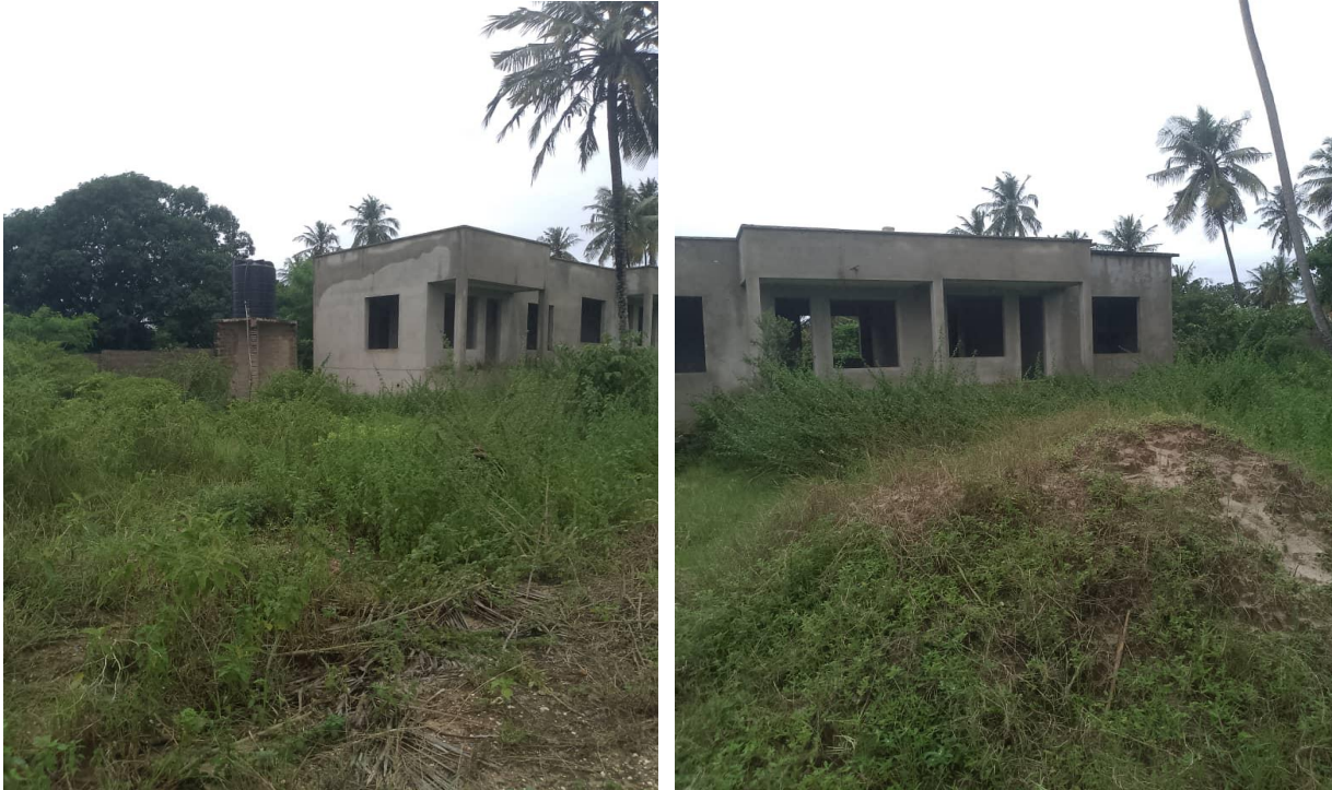
Photo showing the staff houses constructed at site
