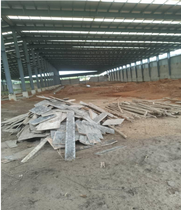
Photo showing the steel columns, beams, trusses and purlins erected at the warehouse buildings.
