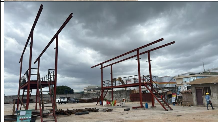
erection of gantry works
