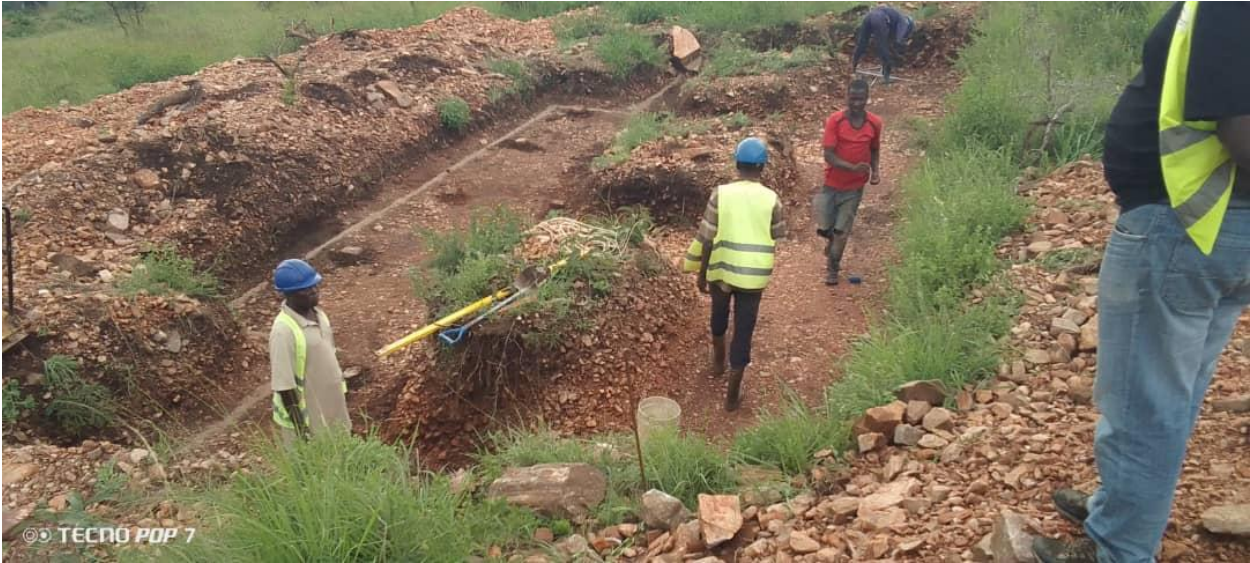
Excavation, foundation and foundation walls for various Staff Quarters
