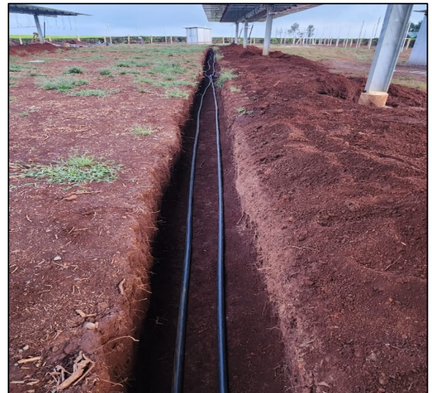
DC Cable Trench of 6 MWp Project in Kenya
