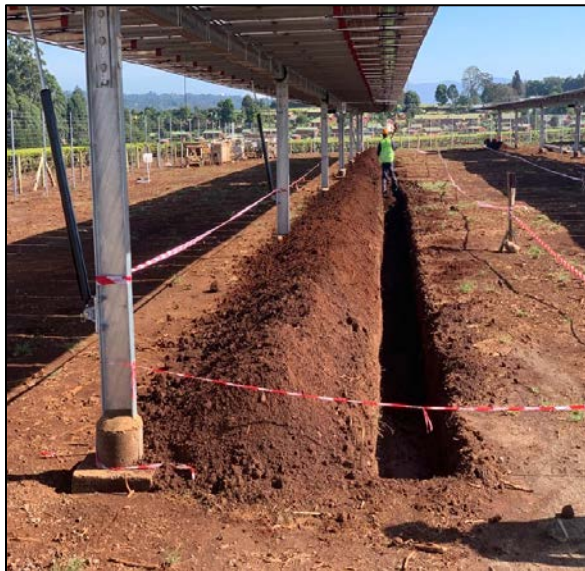
DC Cable Trench of 6 MWp Project in Kenya
