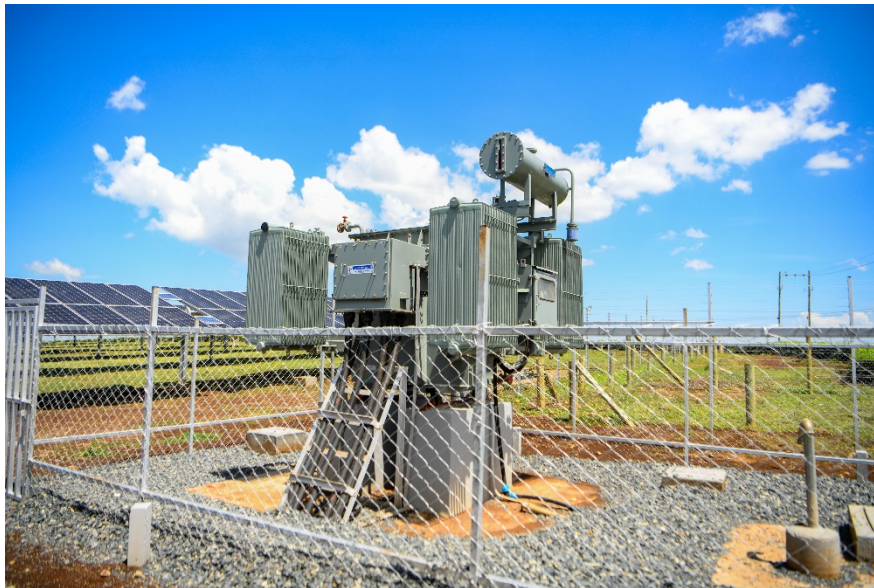
0.415/33 kV Transformer installation by Spenomatic at Finlays Tea, Kenya
