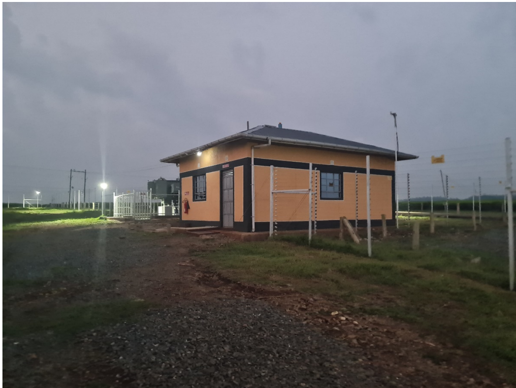
Control Room building at Finlays Project in Kenya
