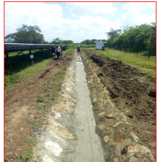
Drainage at 6 MWp done by Spenomatic
