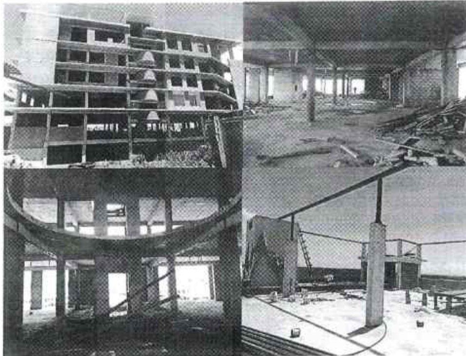
General Overview of the Main Building
