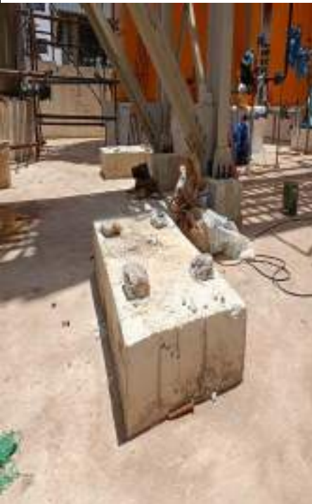
Figure 4- Pump Foundations In Tank form Area- 1.5 Phase
