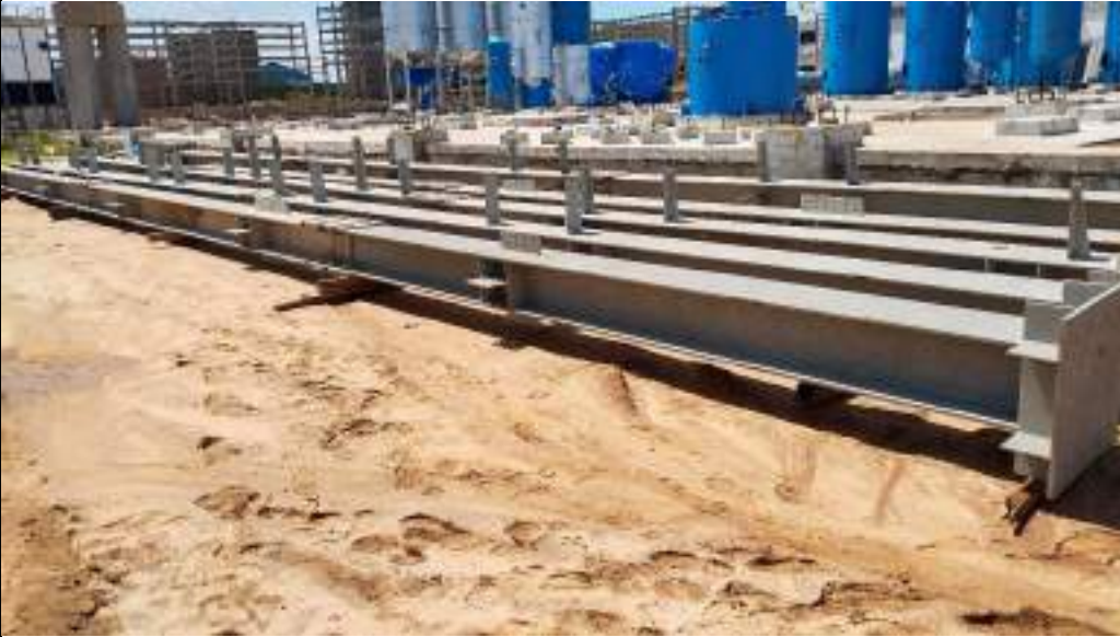
Figure 2-Refinery structure Ground assembly
