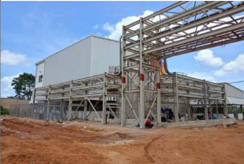
Photo- 1- WTP over all view
