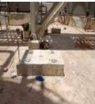
Figure 4- Pump Foundations In Tank form Area- 1.5 Phase
