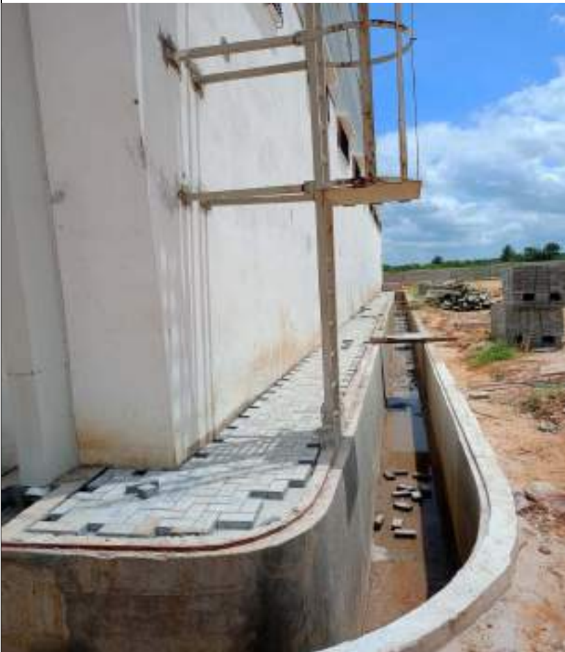
Figure 1: Baving Block work in ware house
