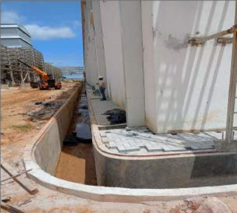
Figure 1: Baving Block work in ware house
