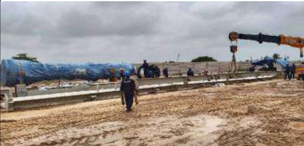
Figure 2-Refinery structure Ground assembly
