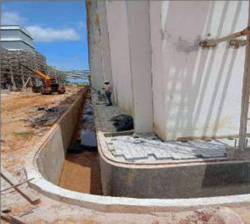
Figure 1: Baving Block work in ware house
