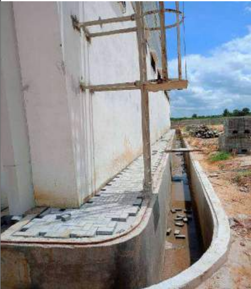
Figure 1: Baving Block work in ware house
