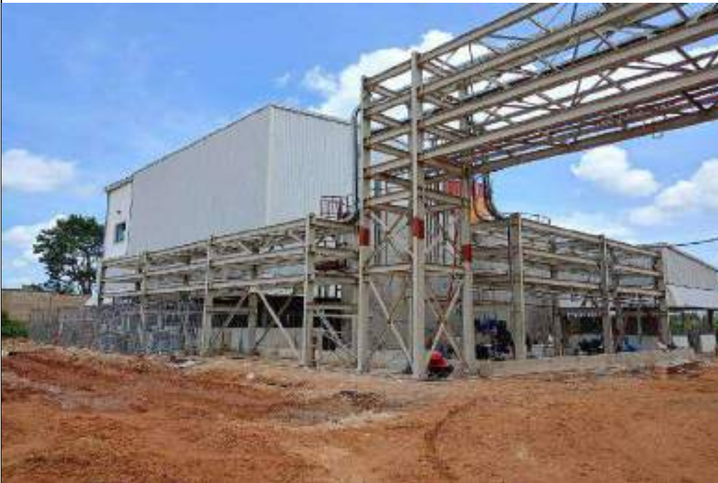
Photo- 1- WTP over all view
