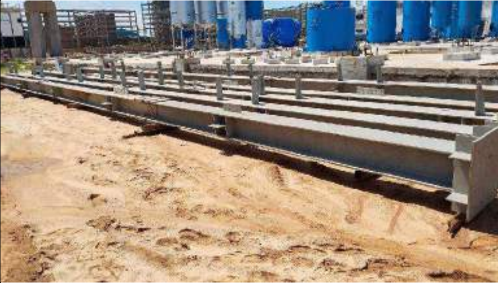
Figure 2-Refinery structure Ground assembly
