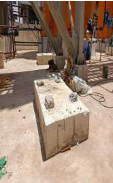
Figure 4- Pump Foundations In Tank form Area- 1.5 Phase
