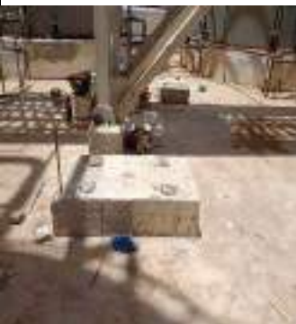
Figure 4- Pump Foundations In Tank form Area- 1.5 Phase
