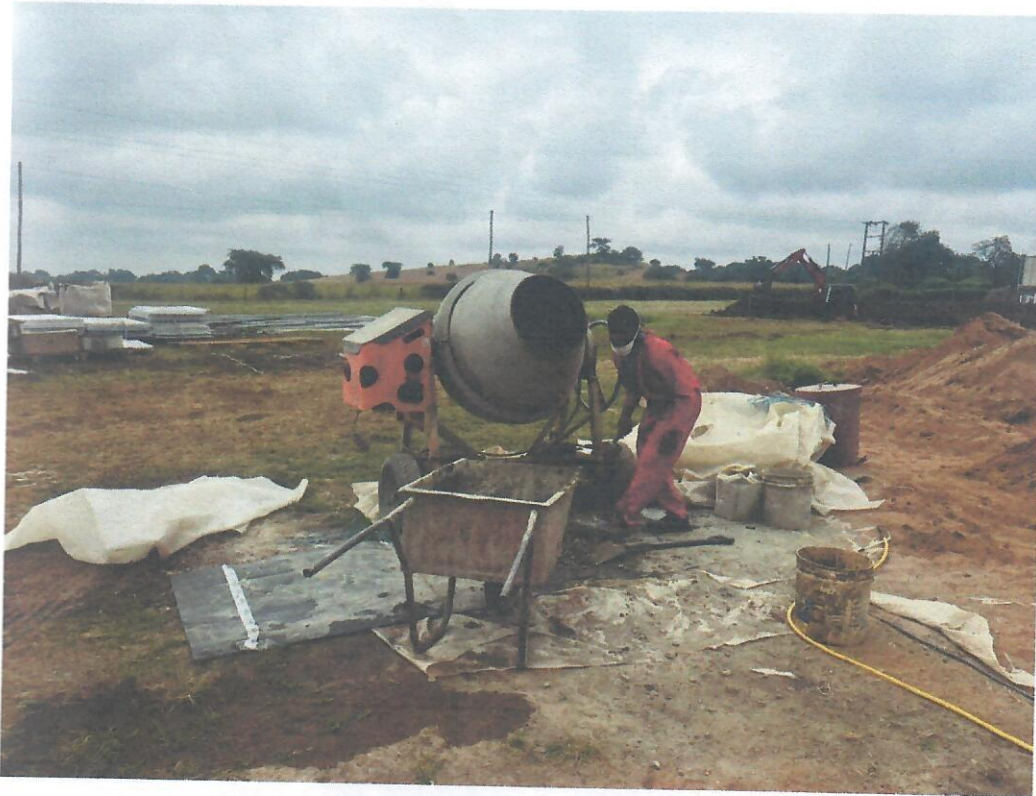
MIXING OF MATERIALS ,SAND AND CEMENT
