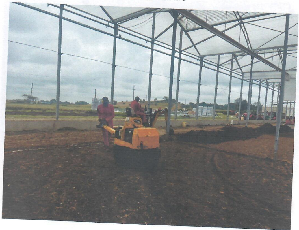
SOIL COMPACTION.
