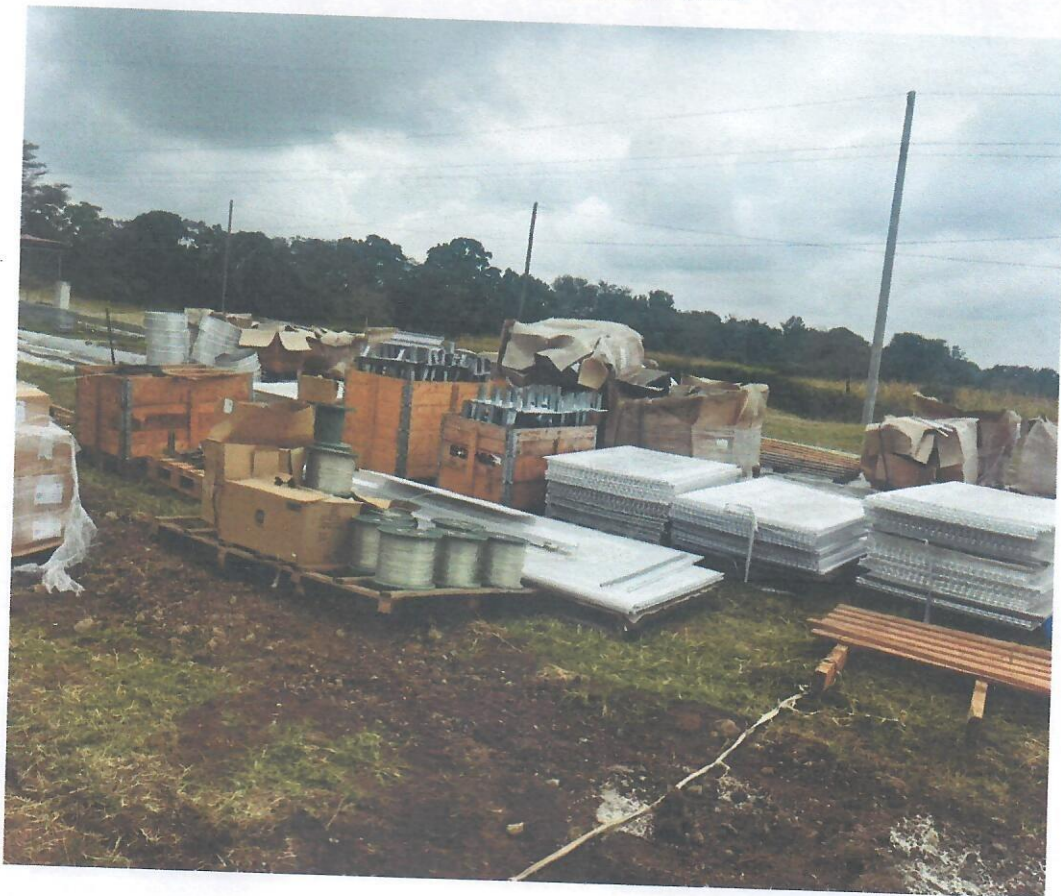
MATERIALS ON SITE
