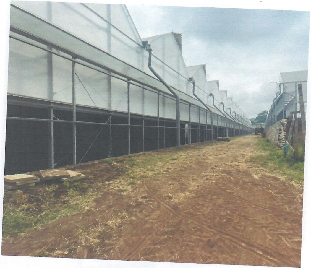
Top Rain Gutters
