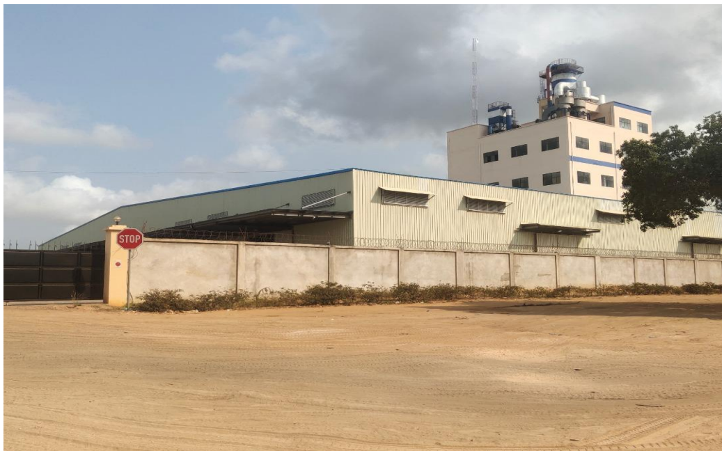
Picture No.2 Outside of the factory
