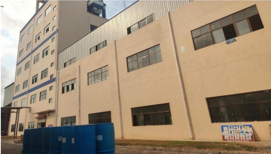
Picture No 1. Outside of the factory
