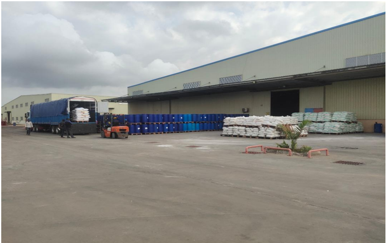
Picture No. 11 Outside Washing powder warehouse
