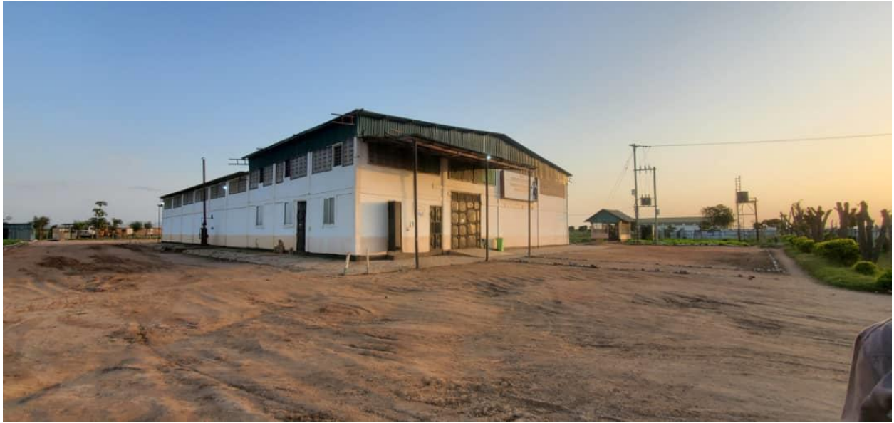
KFS Milling facilities
