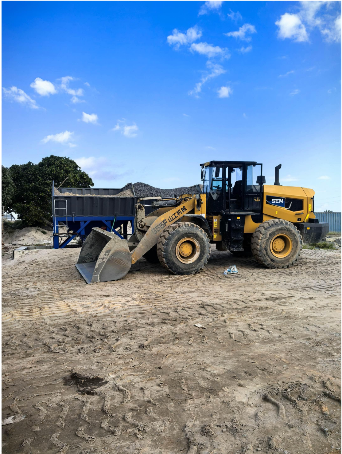
Ongoing excavation and setting out works for the foundation phase.
