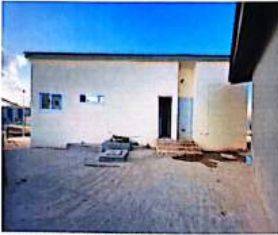
Toilet Block I, General overview Accommodation.
