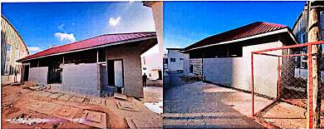
Power House Block, General overview
