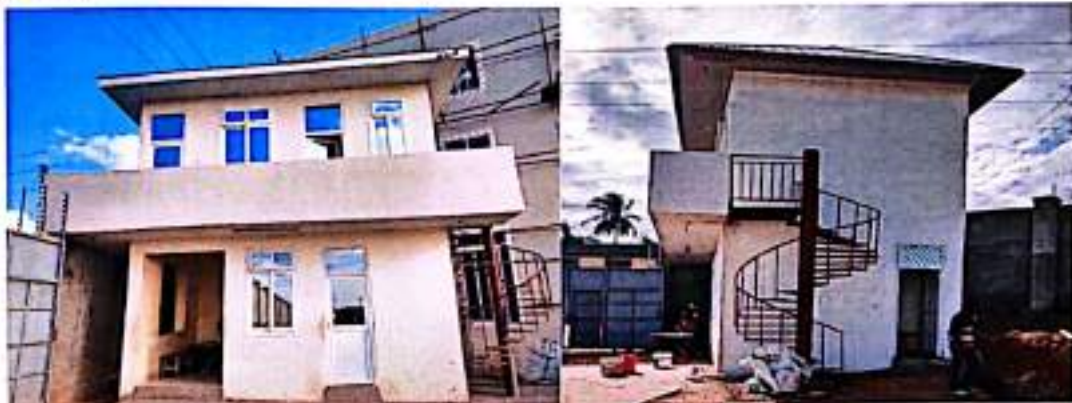
General Overview of the Security Block (Front & Sided Elevation)
