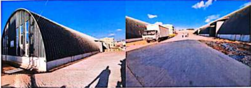
GENERAL VIEW OF MAIN BUILDING
