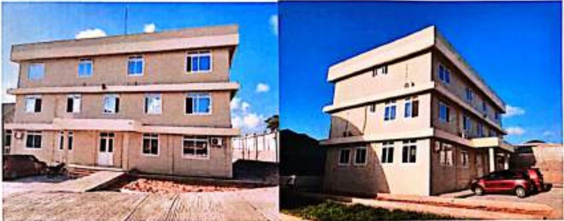
General view of Administration Block, Front and Rear Elevations
