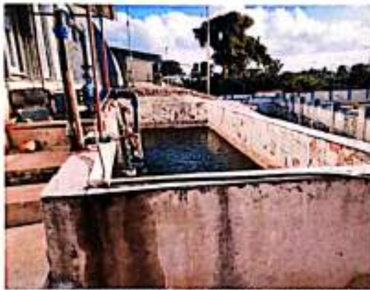
General Overview of the Water Reservoir
