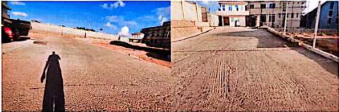
General Overview of the site works improvements (Paved yard)
