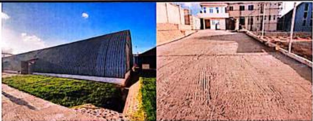
GENERAL VIEW OF SITE WORKS
