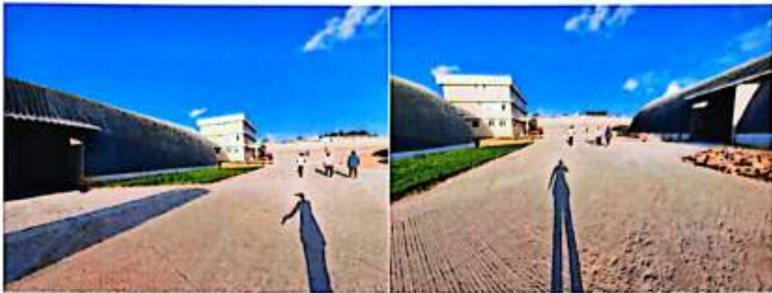
General Overview of the fabricated aluminum profile warehouse I & II Accommodation
