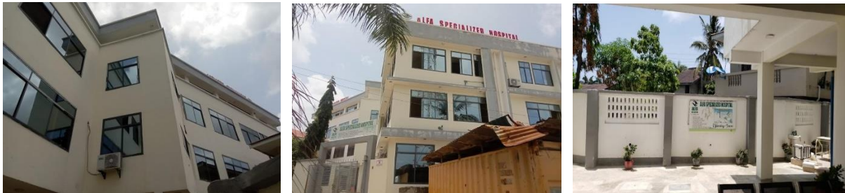
Current exterior overview status of the Hospital Facility main twined 3 storey buildings
