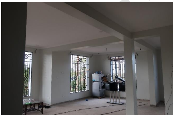
Internal view of the building
