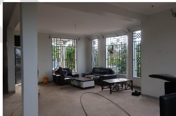
Internal view of the building
