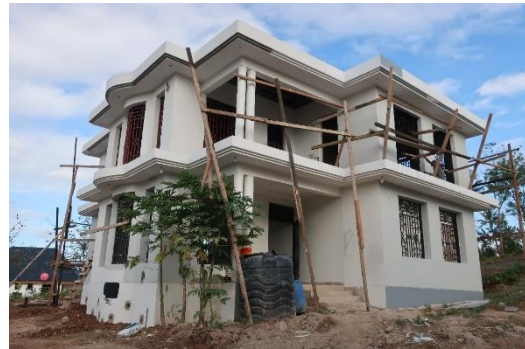
Rear side view of the main building
