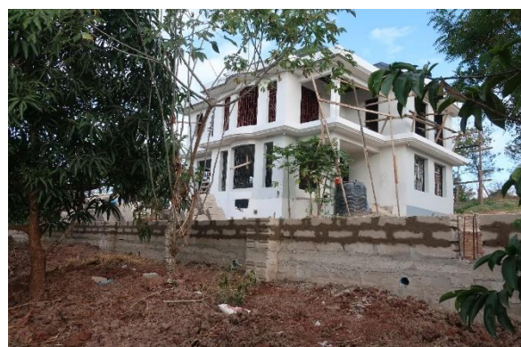
View of site works
