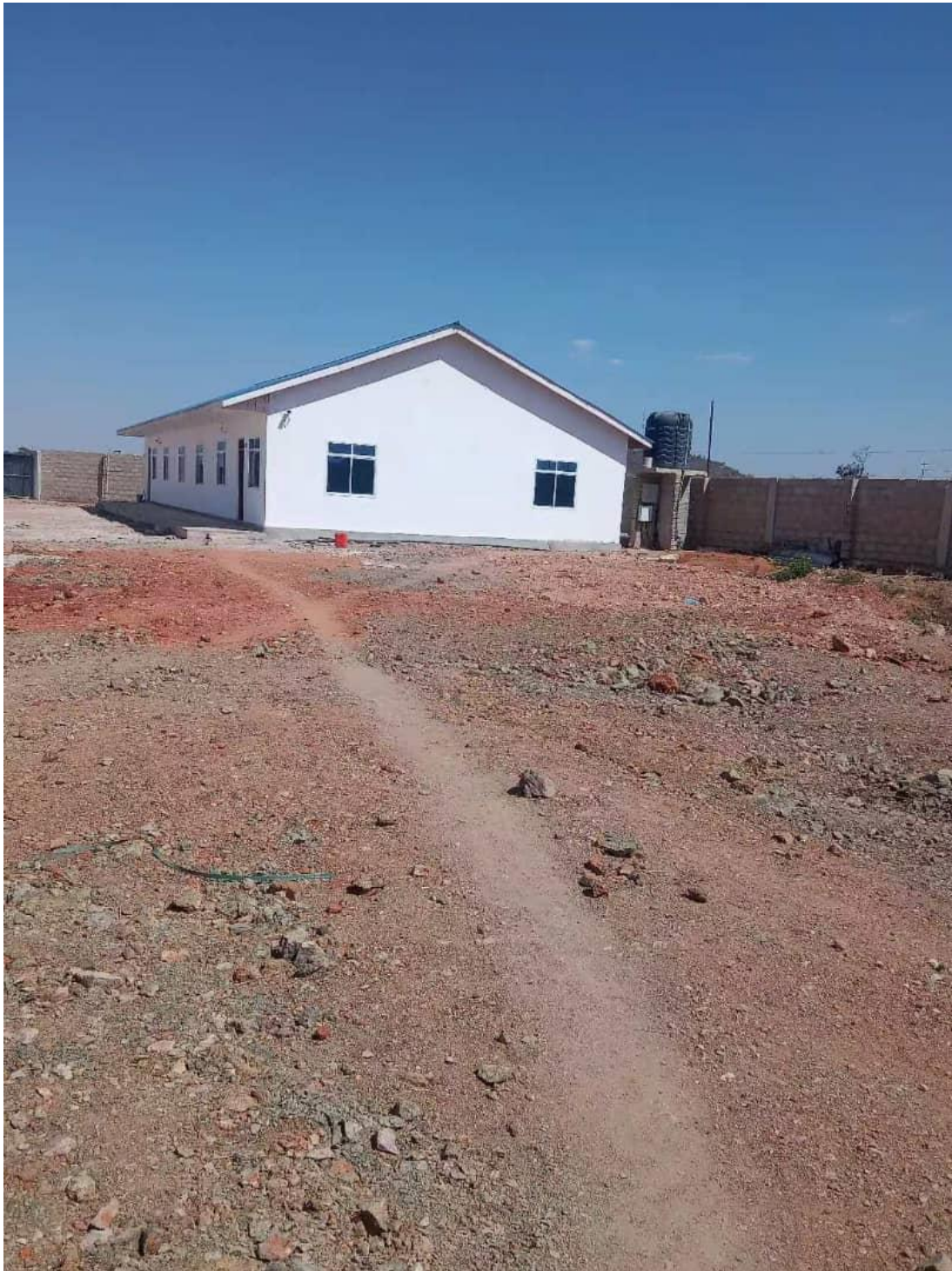
Factory Auxiliary facility with water tank
